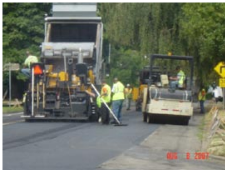
Figure A-5 PDOT crew resurfacing a Portland street
