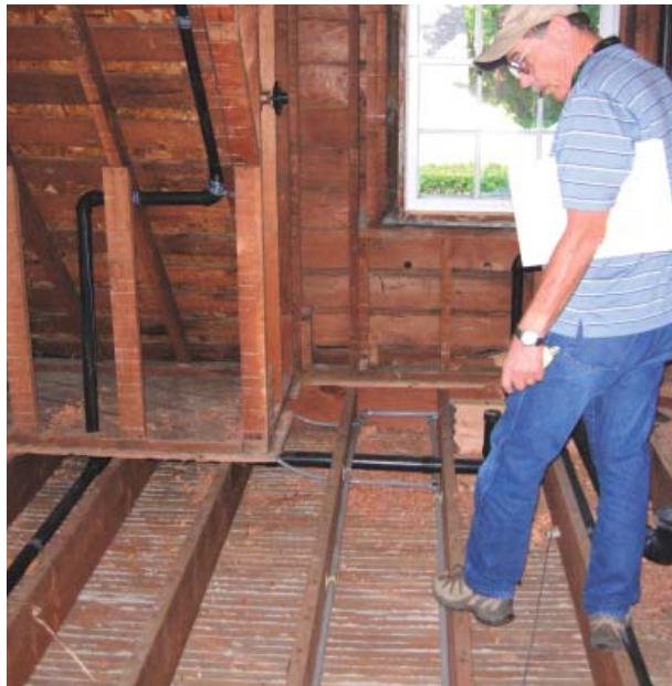
Figure 8 Development Services Inspector
