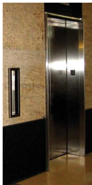
Recessed elevator call buttons were one of the concerns
