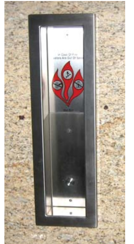
Close up of a recessed elevator call button
