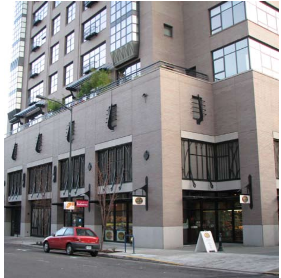
Retail and facade ornamentation on the lower levels of the Elizabeth mask a parking structure, effectively screening views of parked cars and providing an active street environment for the pedestrian.
