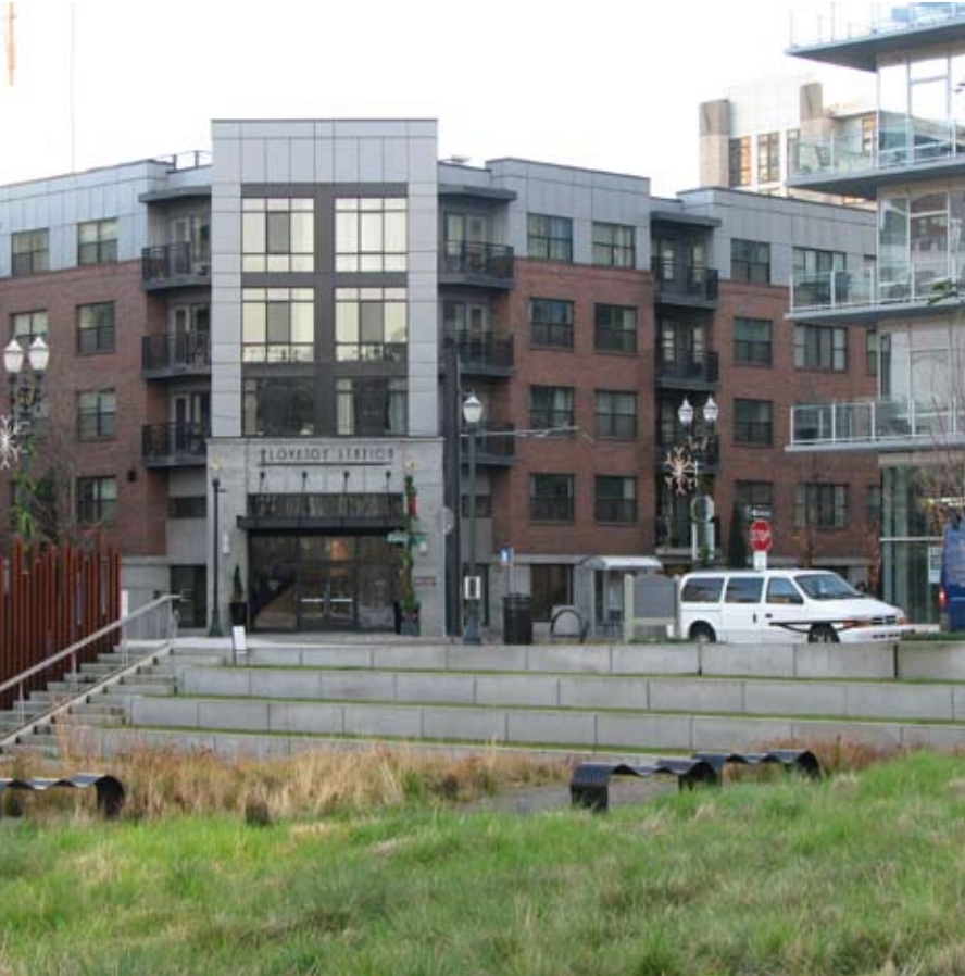
The corner entry and orientation of windows and balconies of the Lovejoy Station apartments formally acknowledges and reflects the significance of Tanner Springs Park.
