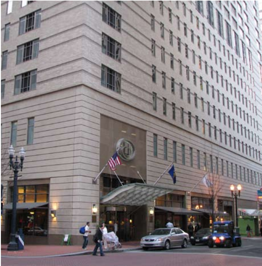
The sloping floors of the parking garage for the Hilton Expansion are masked with the building facade's use of regularly spaced windows that mimic the hotel windows of the floors above.
