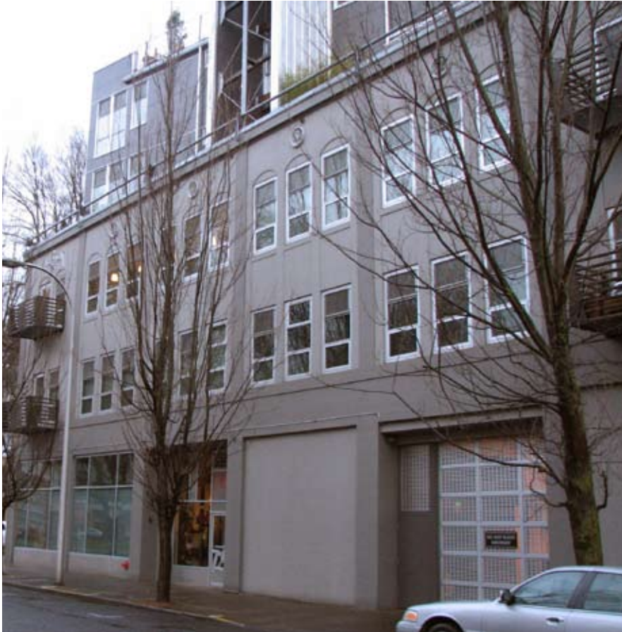
The Flanders Lofts' garage entrance is located along NW Flanders, away from the Park Blocks.
