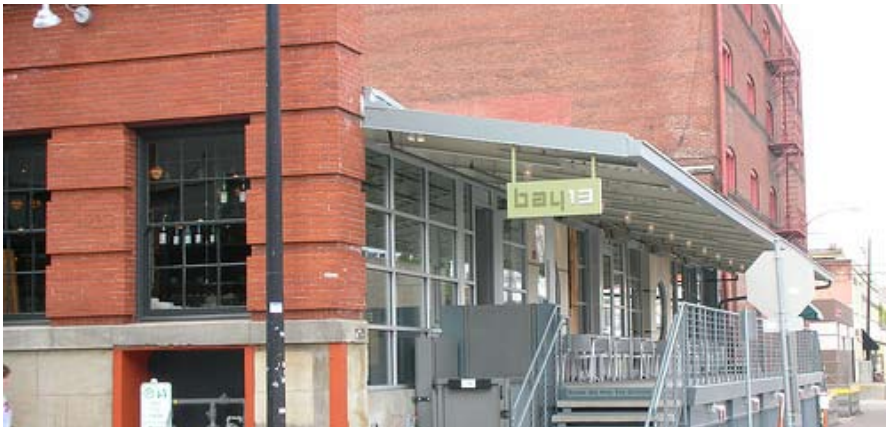
The Avenue Lofts (top) incorporates cobblestone into the pedestrian path where several residential entries front. Bay 13 (bottom), a restaurant located in the historic Crane Warehouse building, has maintained the old warehouse dock, incorporating it into a front entrance.
