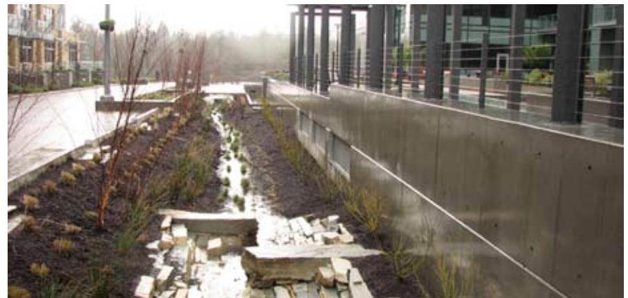
Both the Meriwether (top) and Atwater Place (bottom) include stormwater catchment areas along Pennoyer Street. The design of the landscape allows the areas to serve as both a water feature, landscaped buffer, and critical stormwater function that is attractive with or without water.
