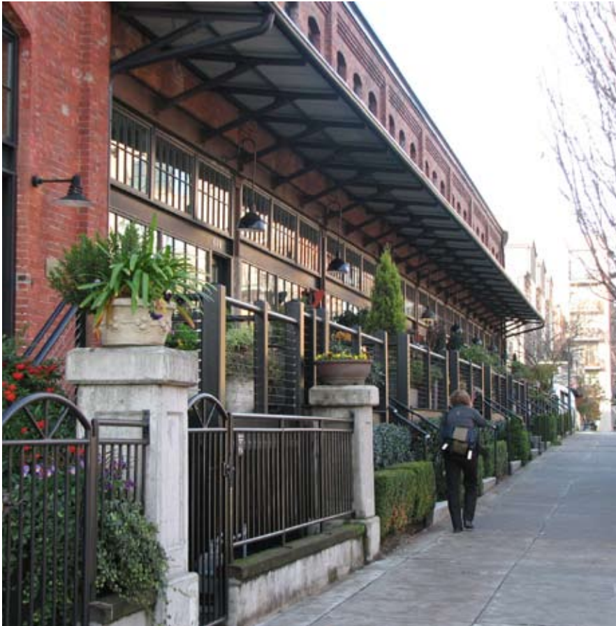
The Pearl Townhouses incorporate railing between private patios and landings which physically separates the public sidewalk and roadway but allows for social interaction.
