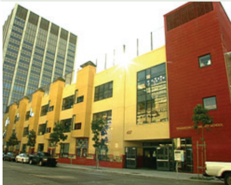
Tenderloin Community Elementary School; San Francisco
