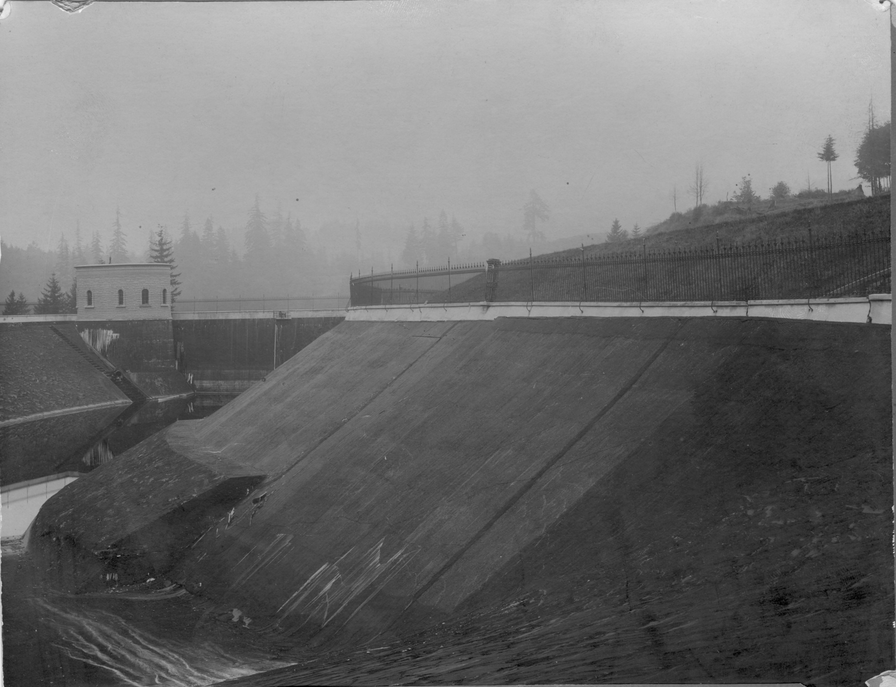
Interior of Reservoir No. 3 showing cracks in lining of West slope. Taken Sept. 28, 1897
