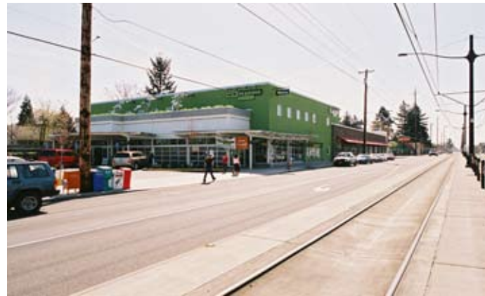
AT PRESCOTT STREET STATION
