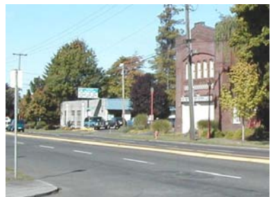
Interstate Firehouse Cultural Center
