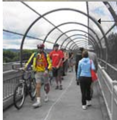
Failing Street Pedestrian Bridge
