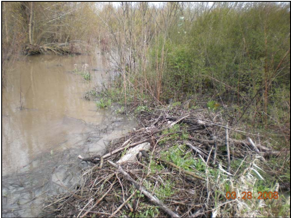
Photo #2 – This photo shows the northern portion of the St. Johns Wetland that is properly functioning. Note the berm and beaver dam that helps to increase inundation.
