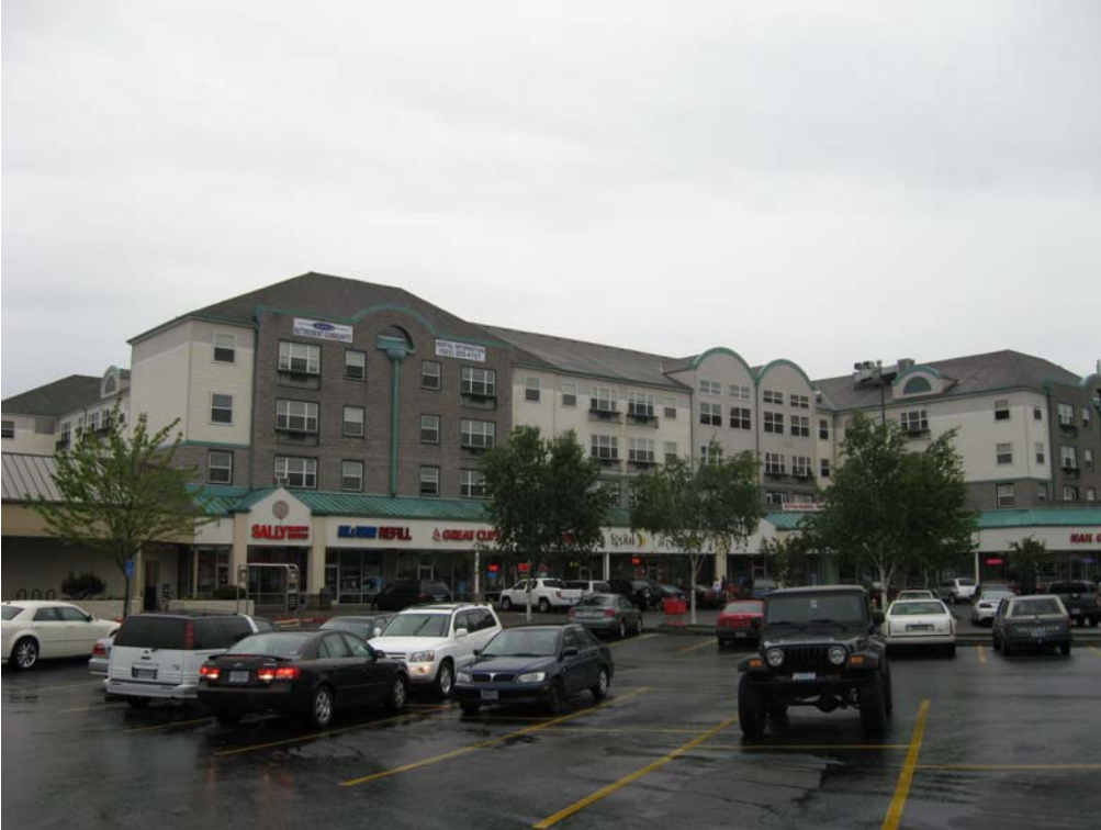
Hazelwood Retirement Community looking southwest from shopping center parking lot.
