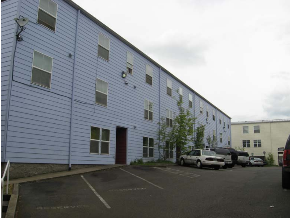
Parking lot looking north at buildings on NE MLK Blvd. and Wygant St.
