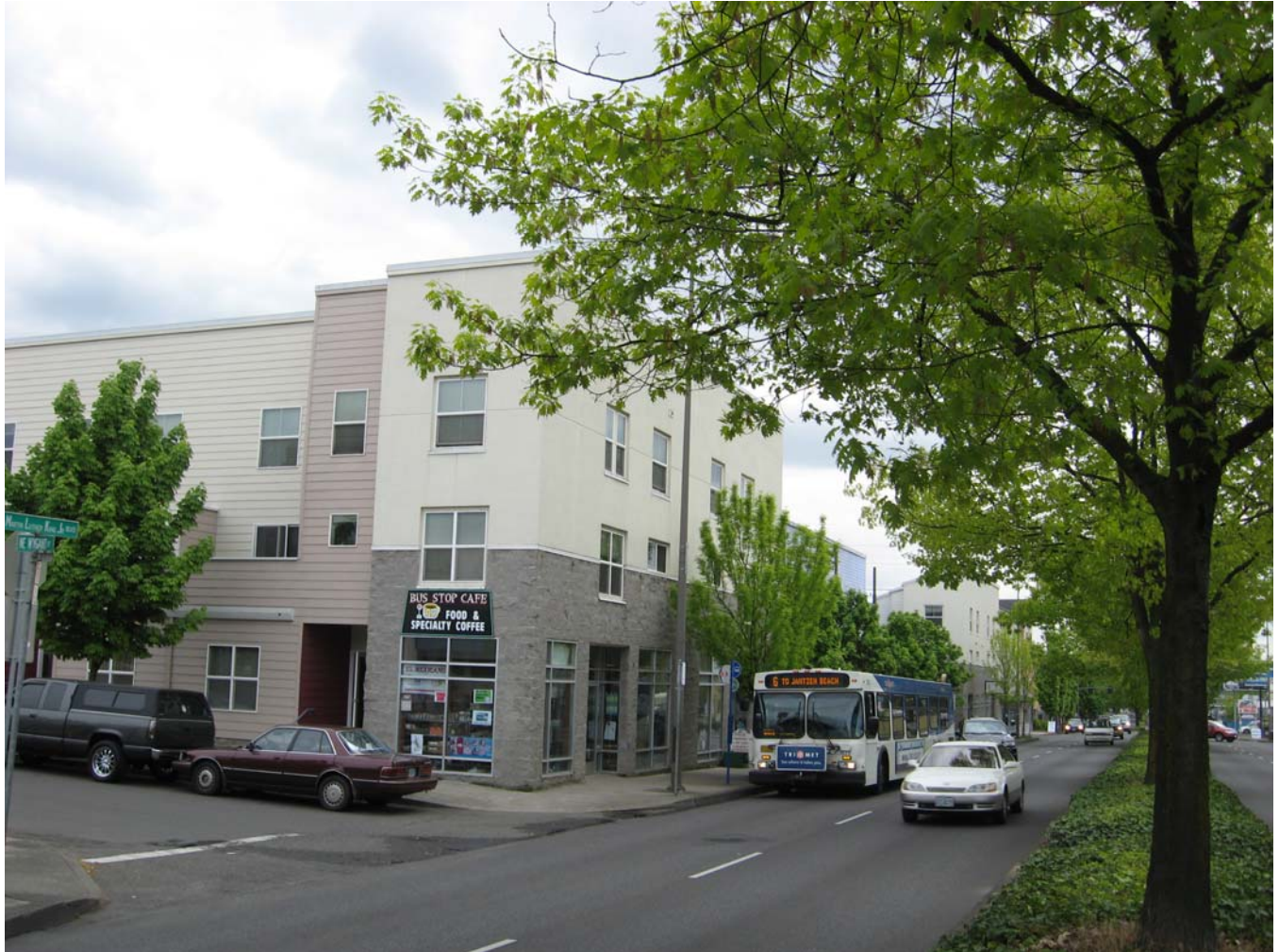
MLK-Wygant Apartments looking south from NE Wygant Street down NE MLK Jr. Blvd.
