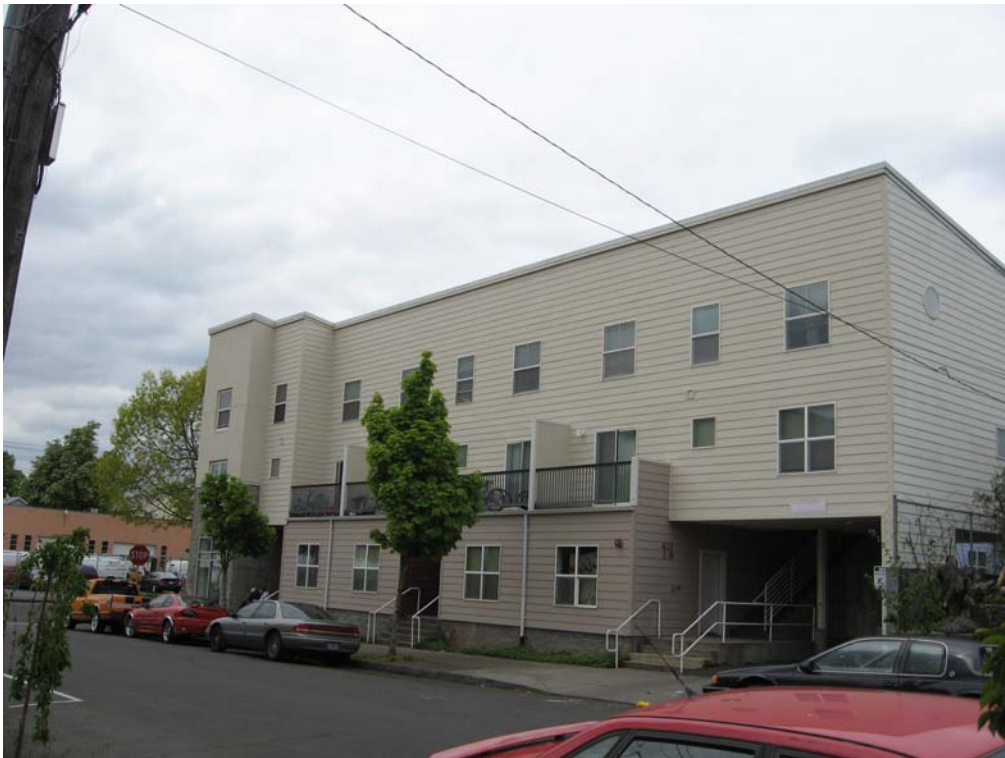
Looking north across Going Street at building on Going.
