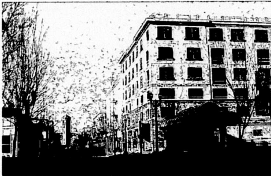
Fifth Avenue Commons Apartments under construction
