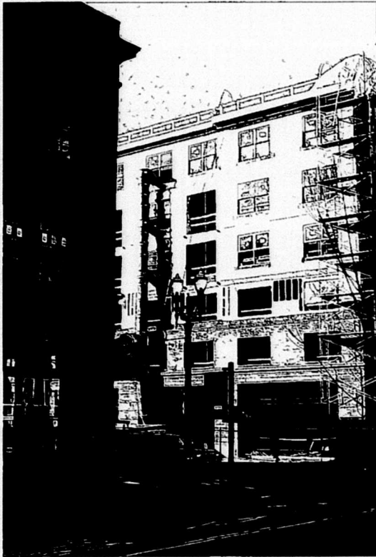
Fifth Avenue Court under construction
