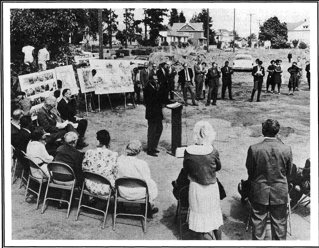
Groundbreaking for Unthank Park-1967 (OHS)
