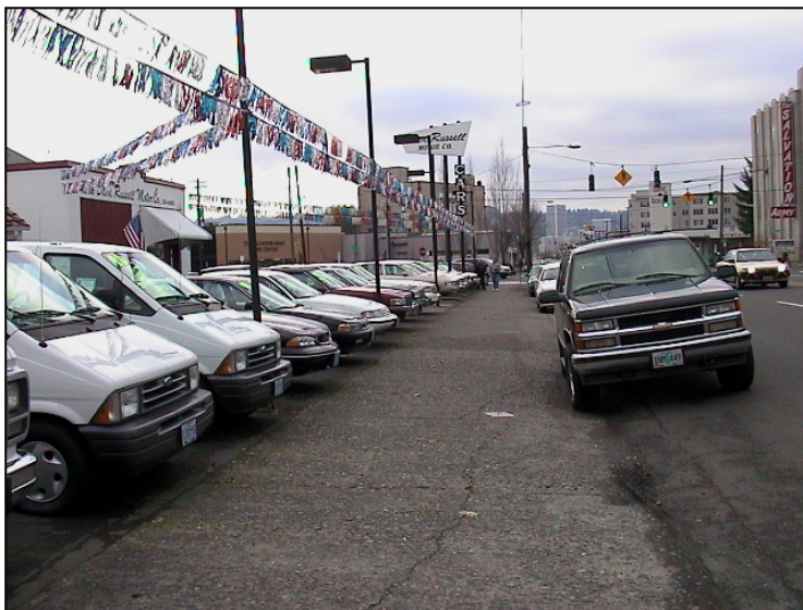
Excess driveways conflict with pedestrian access.
