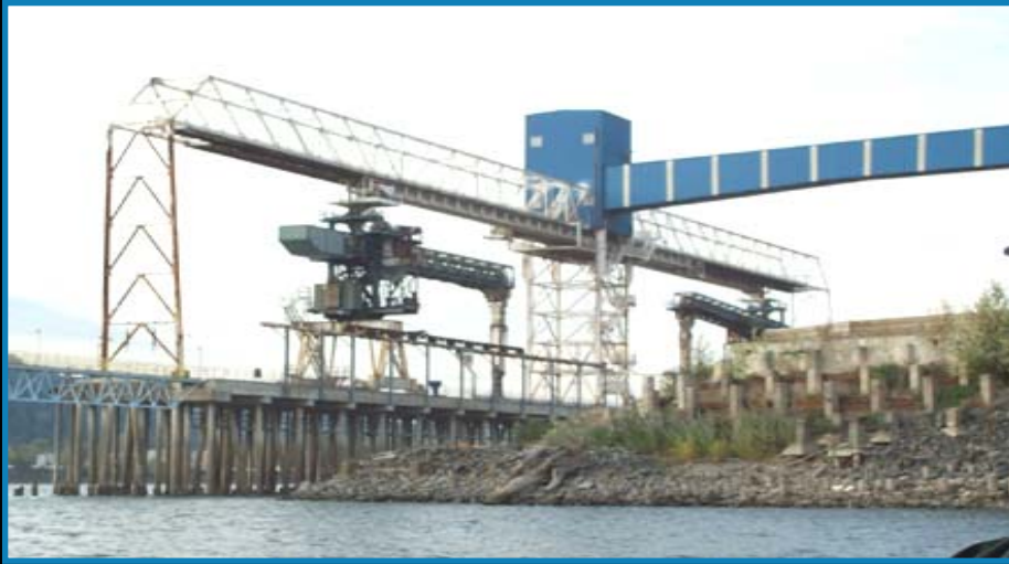
Redevelopment at Terminal 4
