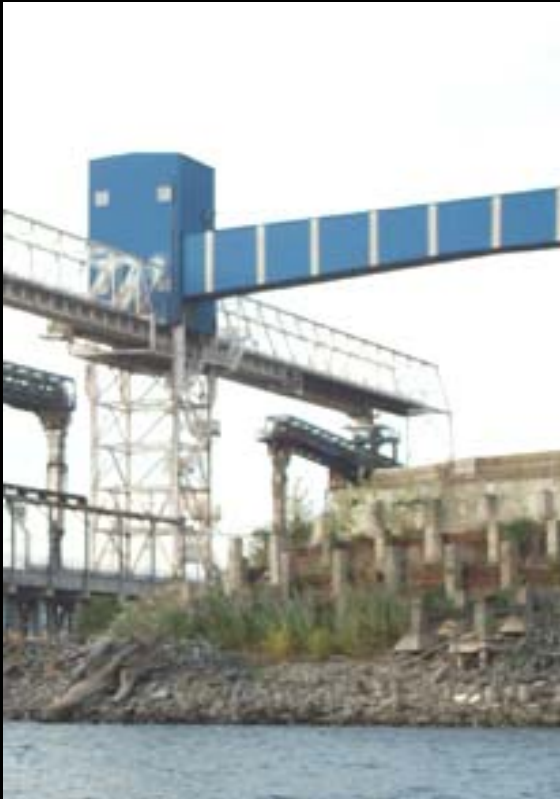
Restored bank at Terminal 4
