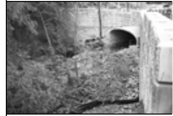
A newly designed intersection improves traffic safety and facilitates fish passage.
