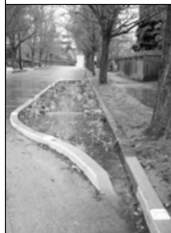
Green Street project at NE Siskiyou and 35th Ave. Street runoff is directed into a landscaped area that filters water and allows it to soak into the ground.
