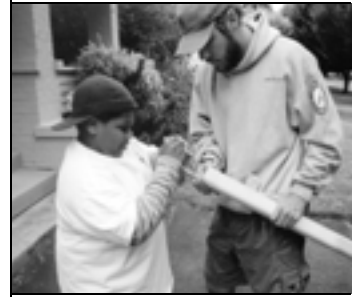
More than 5000 volunteers have helped reduce runoff from household roof drains through the Downspout Disconnection Program.
