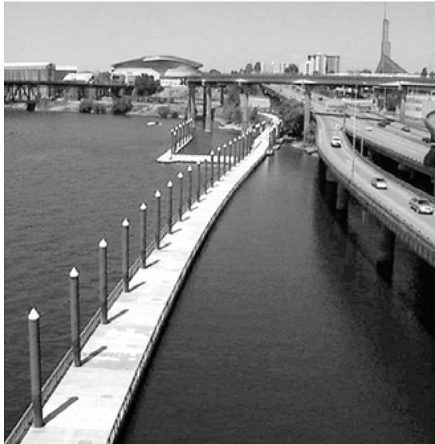
The floating dock of the Eastbank Esplanade allows access next to the I-5 Freeway along the east side of the Willamette River.
