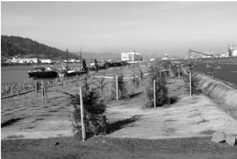
After bank stabilization at Terminal 4
