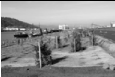
Bank stabilization at the Port of Portland's Terminal 4 incorporated environmentally beneficial features.
