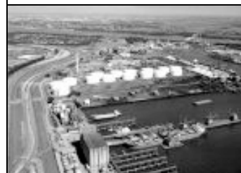
Tank Storage at the Port of Rotterdam
