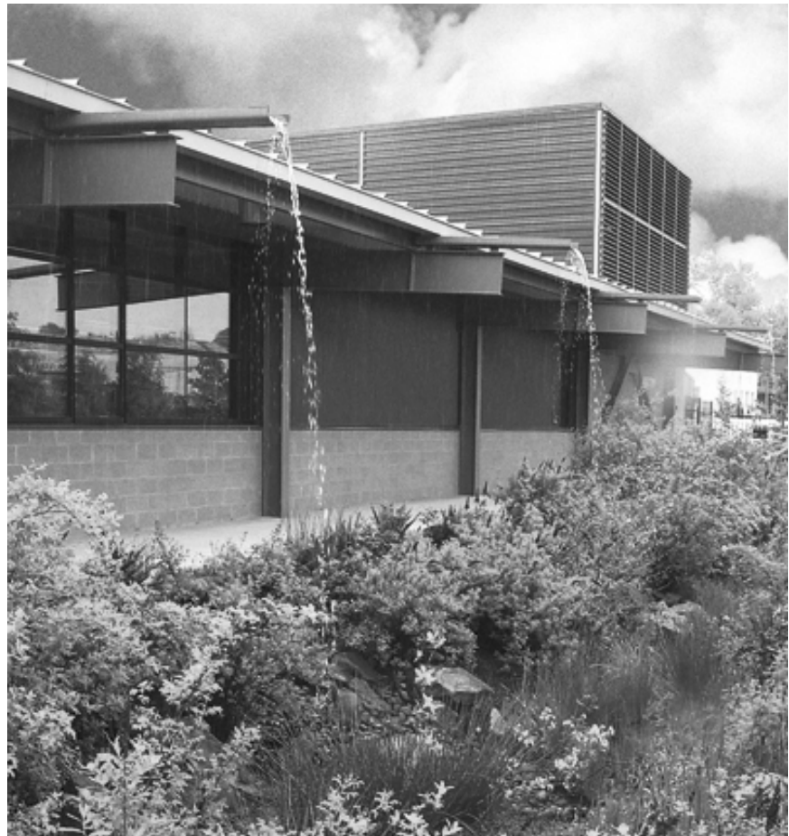
The Bureau of Environmental Services Water Pollution Control Lab captures rainwater and directs it to a bioswale.
