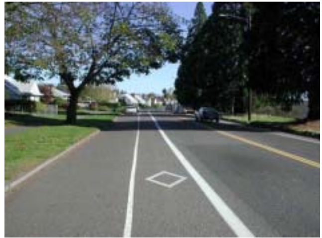
Willamette Blvd. looking east from the University of Portland
