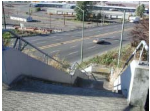
Stairways offer the only direct access from N. Greeley
