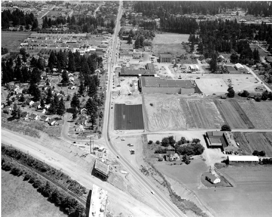
View east along NE Halsey. Both Fred Meyer, in the middle, and the I-84 Freeway, in the foreground, are under construction, probably the mid-1950s. Courtesy of Bob Earnest
