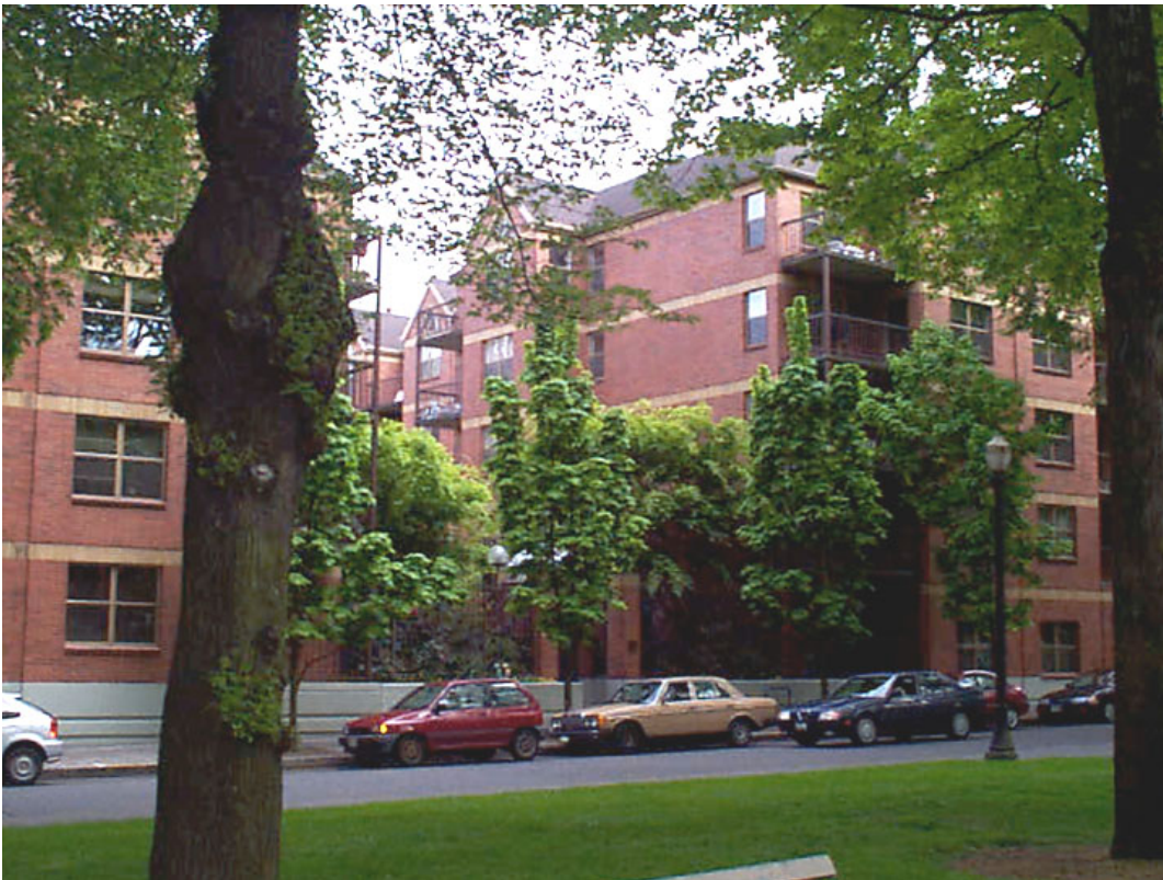
South Park Square Apartment complex on the Park Blocks in downtown Portland
