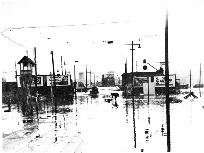
East side approach to Morrison Street Bridge, Portland.
