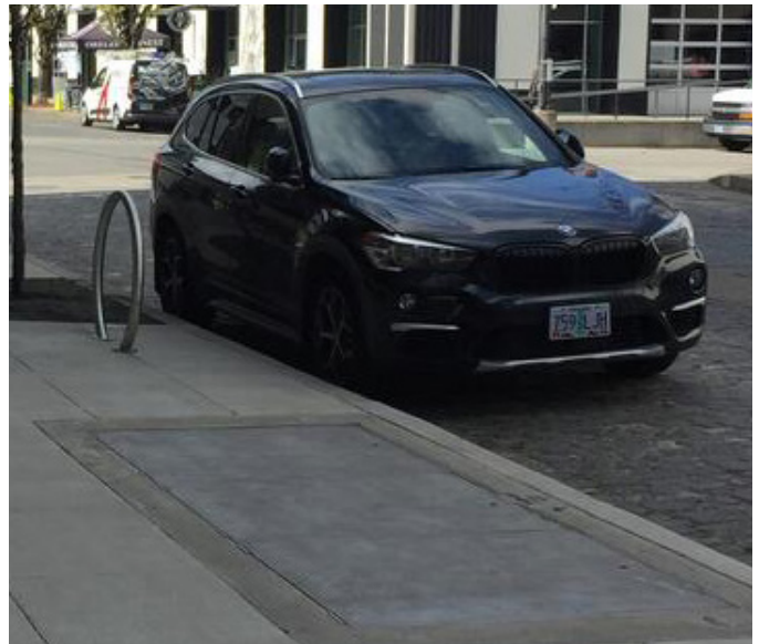
Figure B-17: Hatch/utility vault covers should be located in the Furnishing Zone. Covers located in the Pedestrian Through Zone can effectively narrow the Pedestrian Through Zone as people walk around them to avoid walking on lids.
