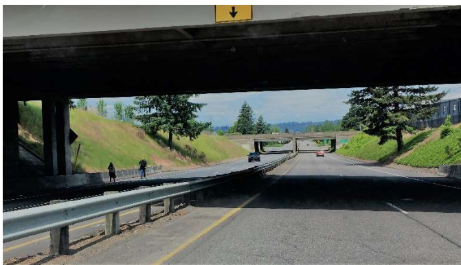
People walking on 82nd Avenue/Highway 213, near the Killingsworth overpass, in the airport segment of the corridor. Pedestrian environment here is unsafe. Companion to this study, PBOT's 82 nd Avenue Study includes safety improvements for people walking—often to access jobs—in this part of the corridor.
