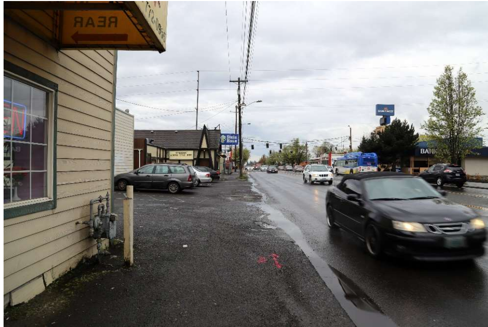
Blacktop offers ambiguous pedestrian path and blends with the roadway. There is no noticeable separation of material and/or vertical plane between the pedestrian zone and vehicles lanes.
