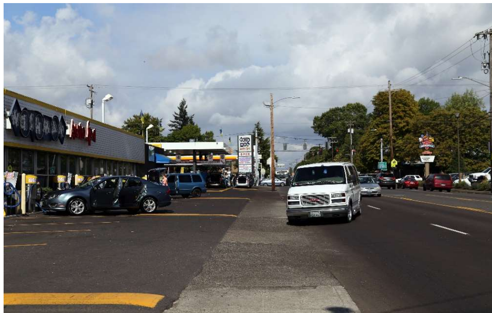
Long curb cut at the Washman Auto Spa. This is anticipated to be remedied at the same time with improvements to the property.
