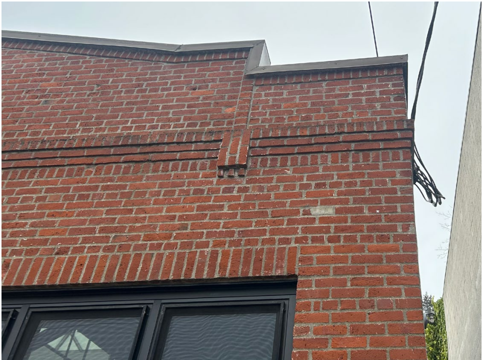
Sydney Wallace building - Soldier course at cornice and window head, metal parapet cap, and corbeling detail. Body of building is a modified English Bond.
