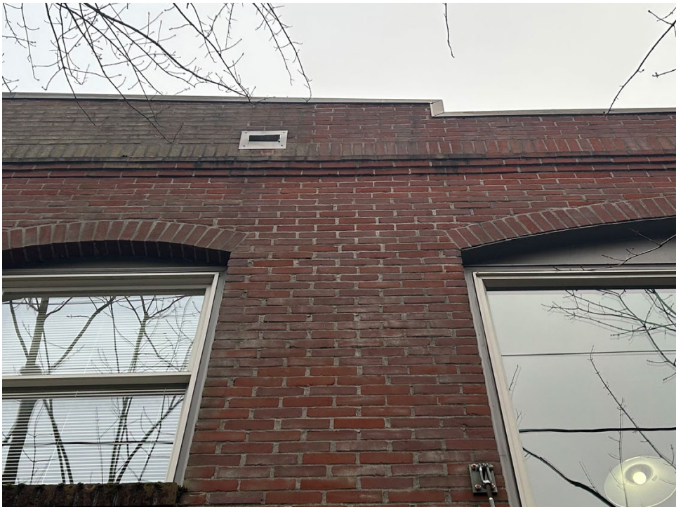
3015 SW 1st Ave "Loft" - Soldier course at window head and corbel, metal parapet cap, and corbeling detail. Body of building is a Running Bond.
