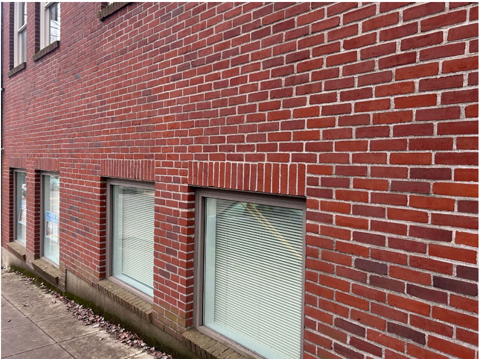
3015 SW 1st Ave "Loft" - Soldier course at window head, brick sill, and stepped concrete foundation wall.
