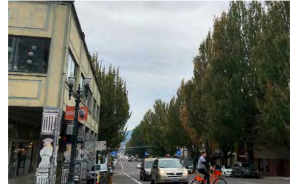
The arcades on Burnside Street are a unique placemaking design feature not found elsewhere in the City.
