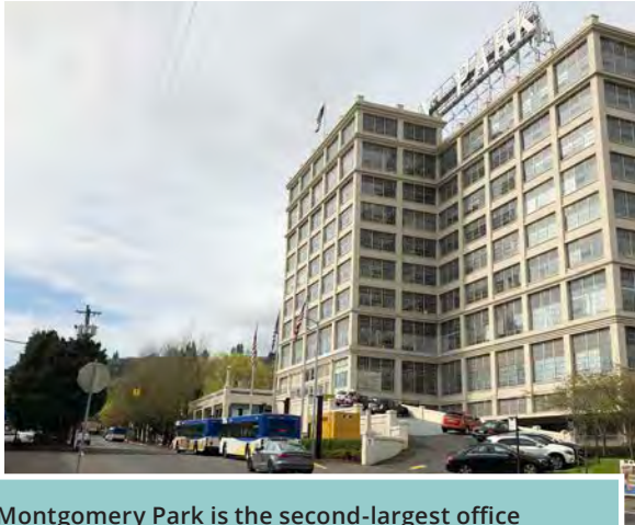
Montgomery Park is the second-largest office building in Portland, hosting a variety of businesses and services.
