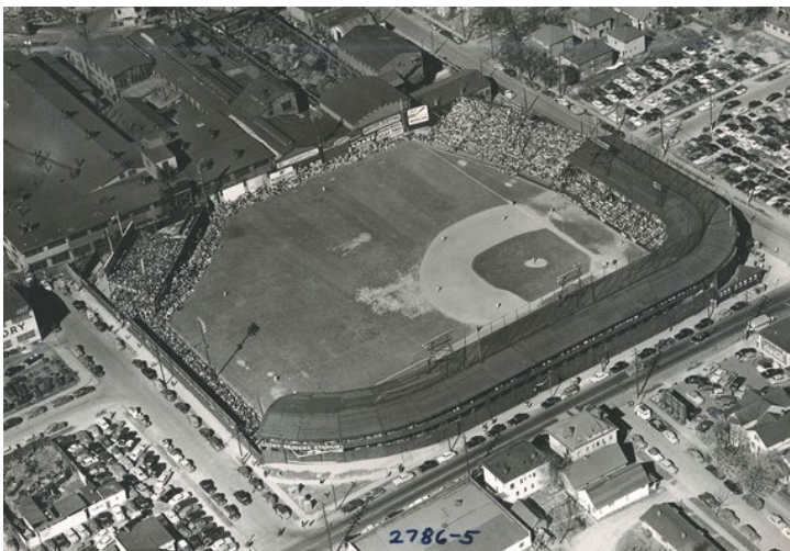
Vaugh Street Park, 1951
