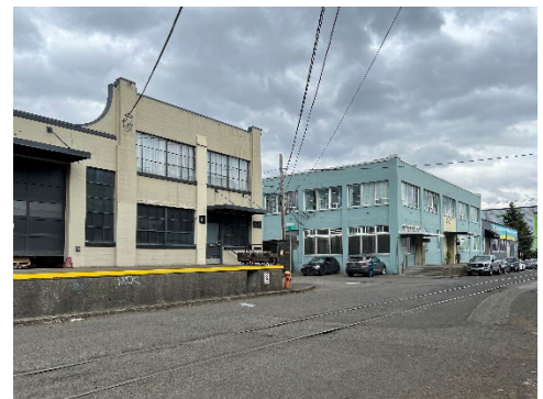
Existing dock conditions on NW York Street
