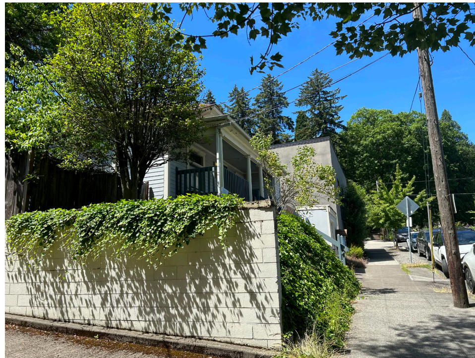
B) 118 SW Porter St retaining wall- Facing Southwest
