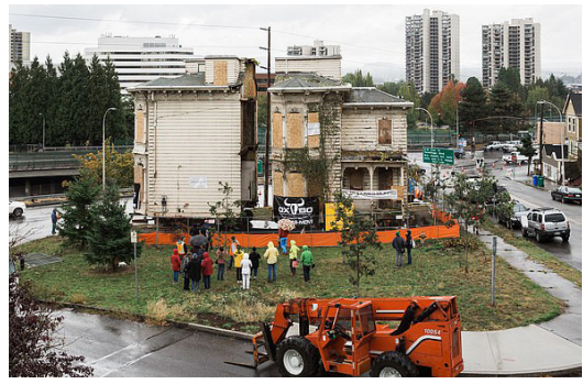
Photos of Fried-Durkheimer House relocation
