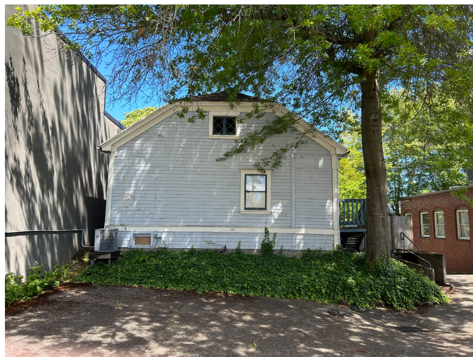
D) Existing on-site Parking / Back of 118 SW Porter property - Facing North
