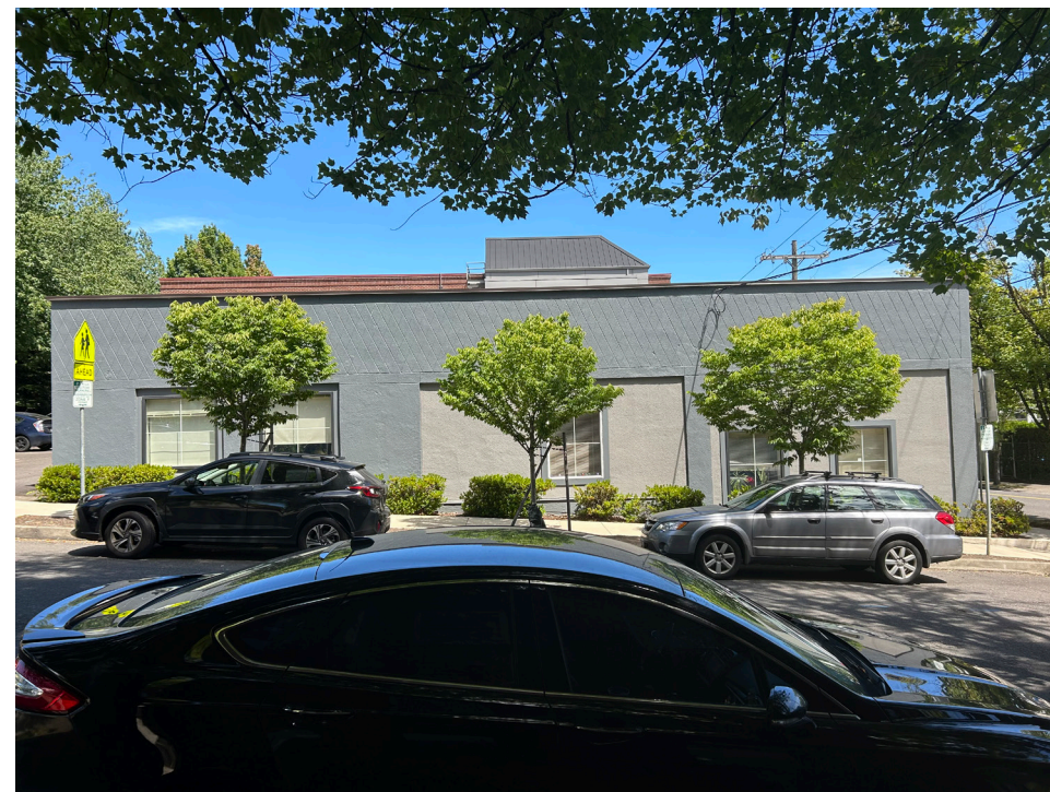
D) Porter Street Frontage - Facing North
