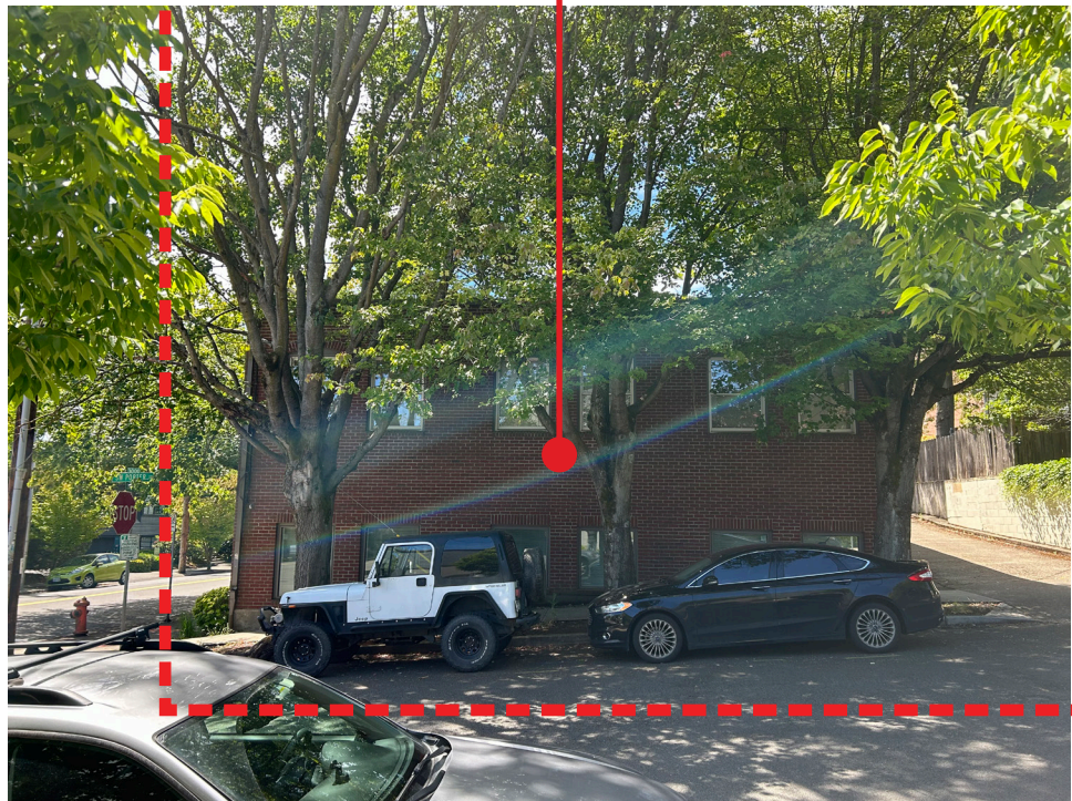
A) Porter Street Frontage - Facing South
