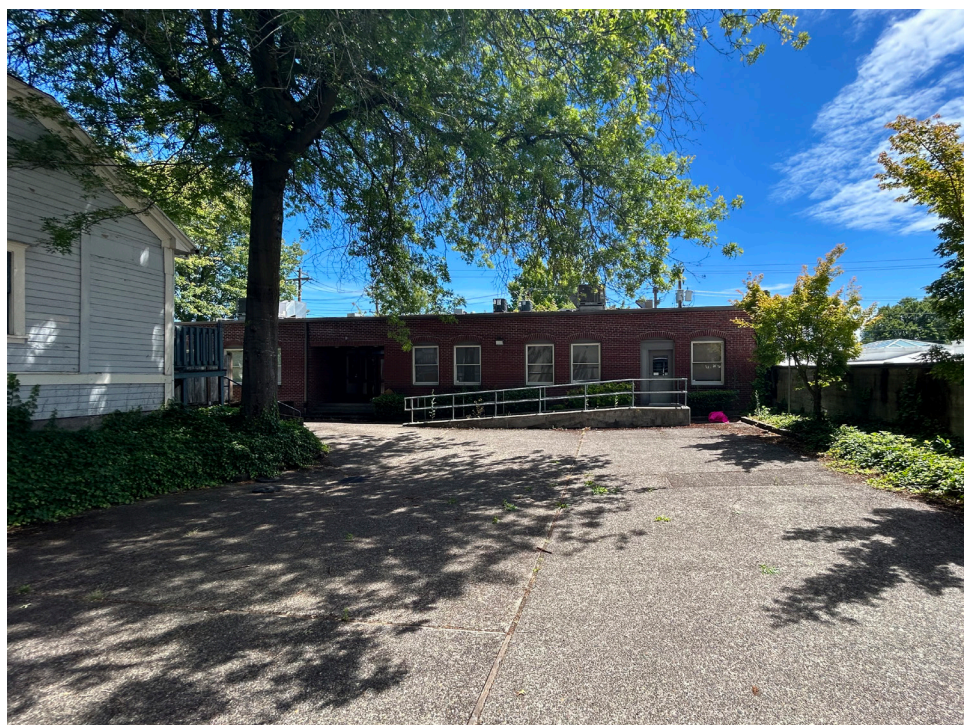
C) Existing on-site Parking - Facing East
