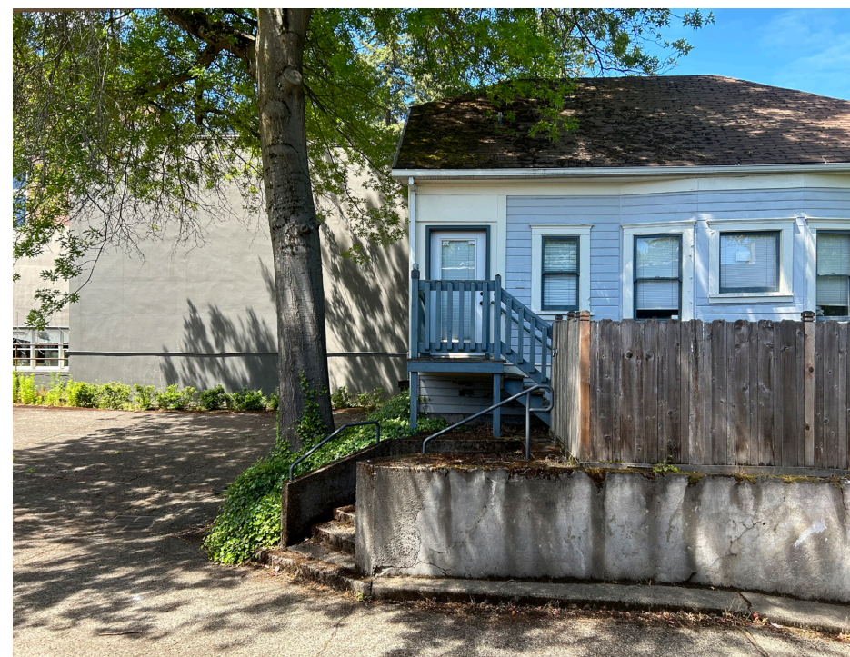
C) 118 SW Porter St - Facing West
