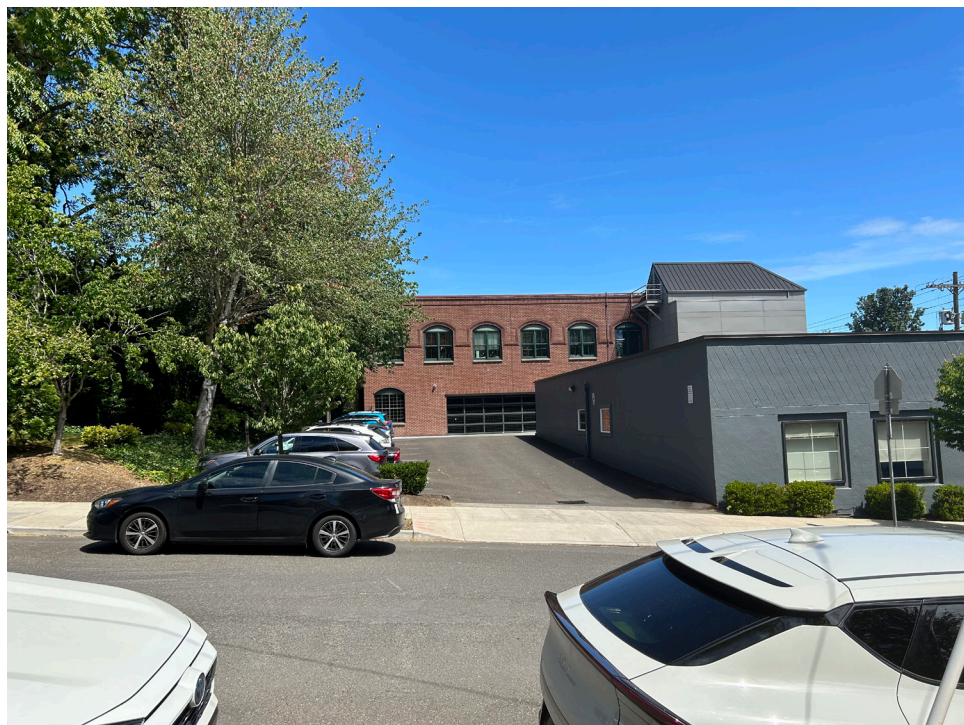
C) Porter Street Frontage - Facing North
