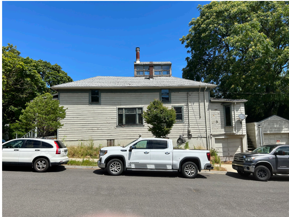
A) Porter Street Frontage - Facing North
