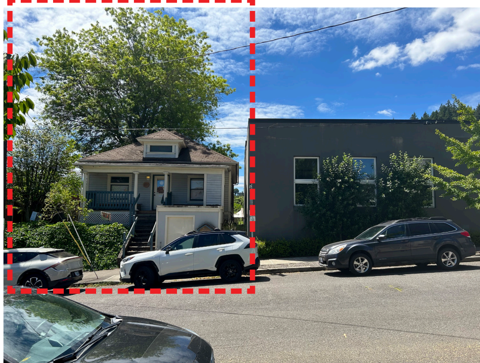
C) Porter Street Frontage - Facing South
