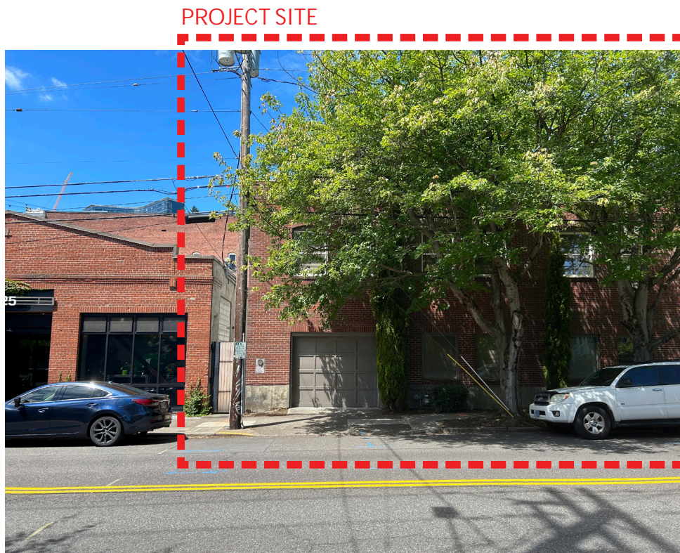
C) SW 1st Ave. Frontage - Facing West
