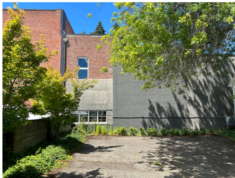
D) Existing on-site Parking - Facing West
