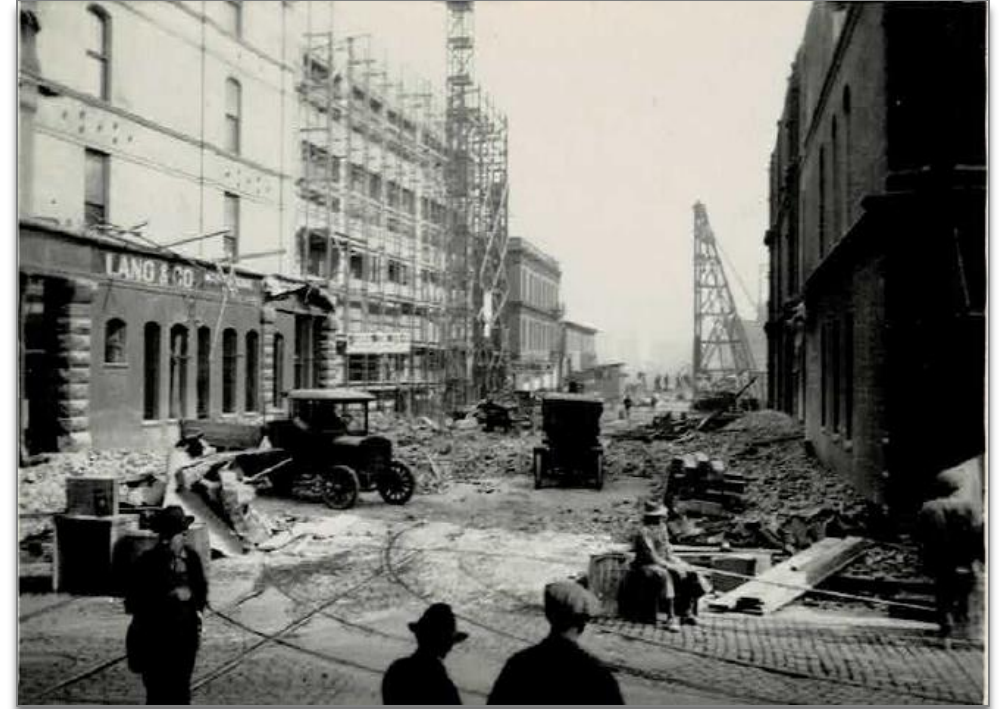
Tent and Awning Co Building façade removal Steve Dotterer Collection
