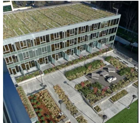
Building with eco roof and raised courtyard
