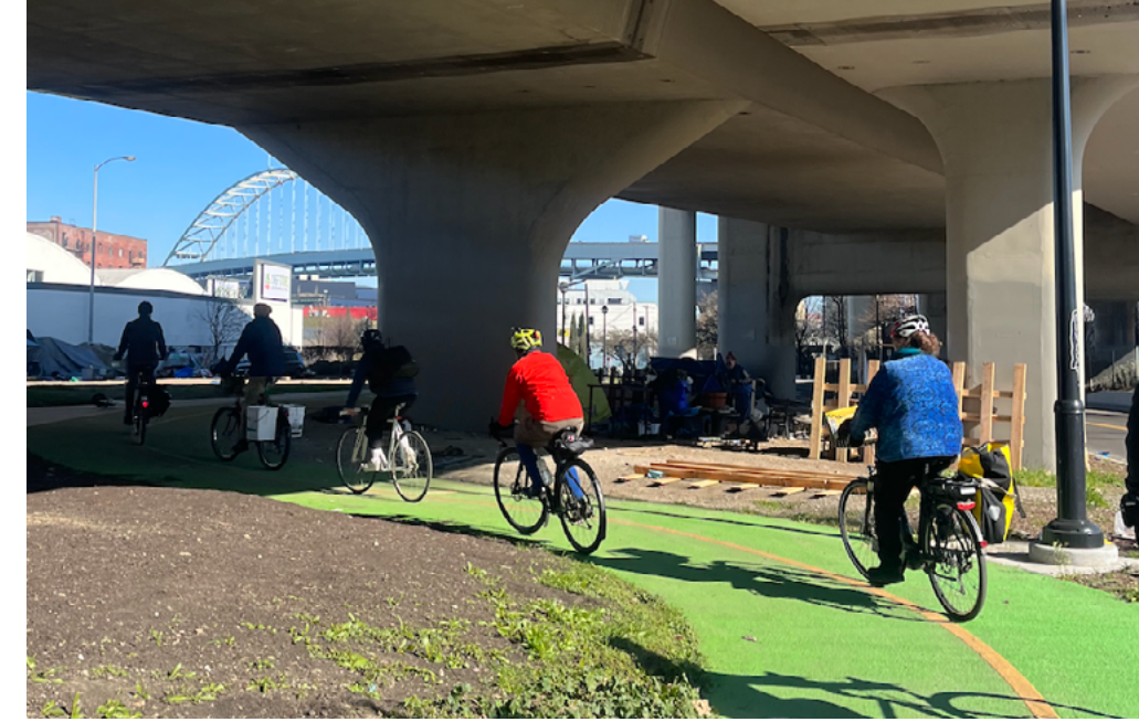
An LID funded the extensions of NW 20th Avenue and NW Thurman Street in Northwest Portland, reconnecting the street grid under US-30.
