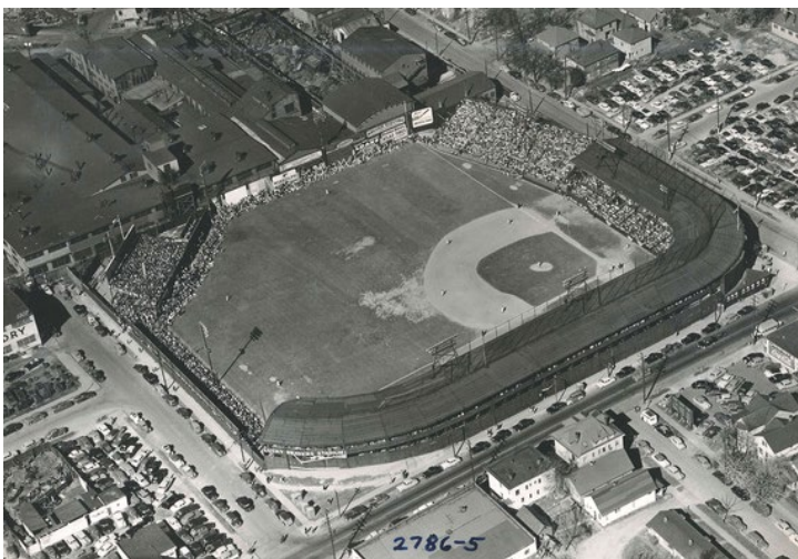
Vaugh Street Park, 1951
