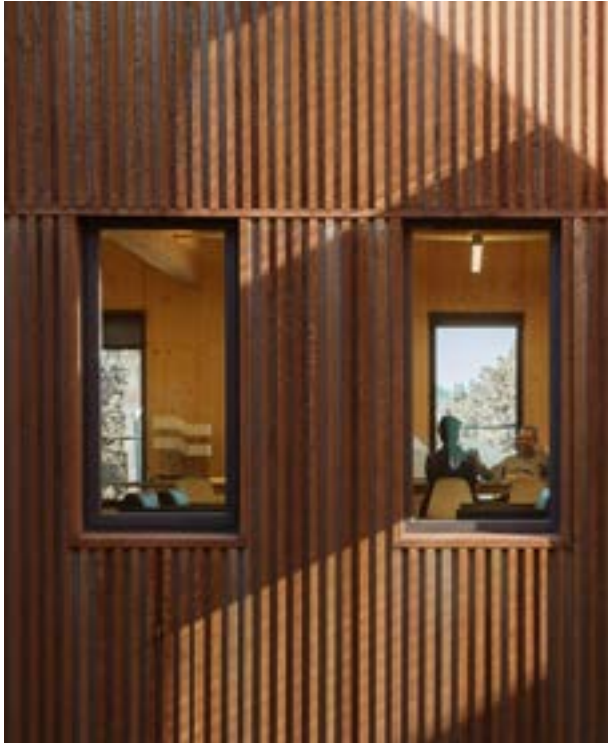
CORRUGATED METAL SIDING
