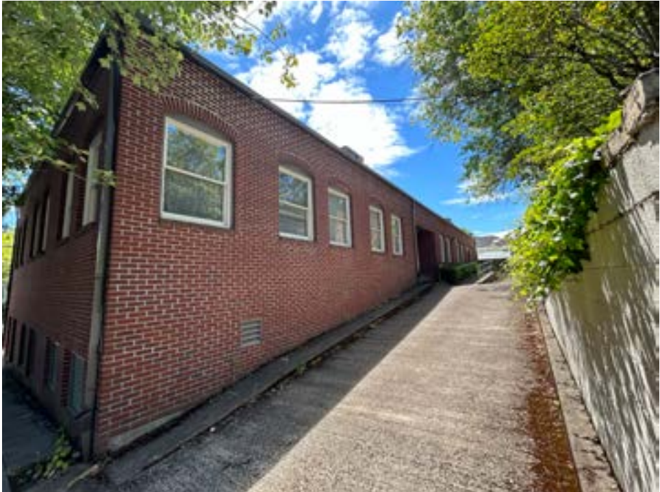
A) Existing on-site Parking Access - Facing South
