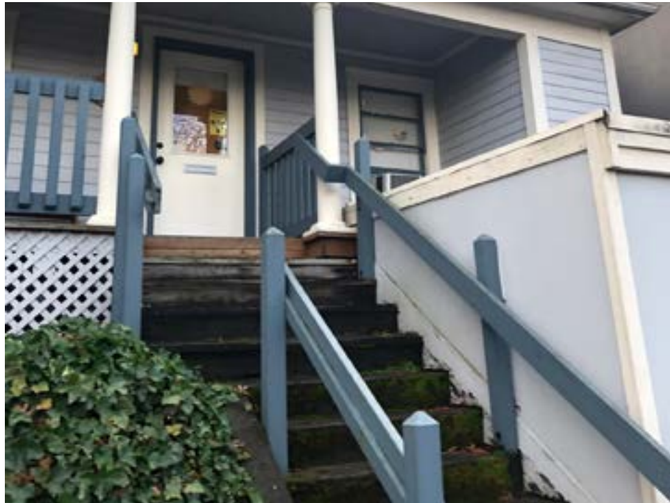
A) 118 SW Porter St - Front porch and steps - Facing South
