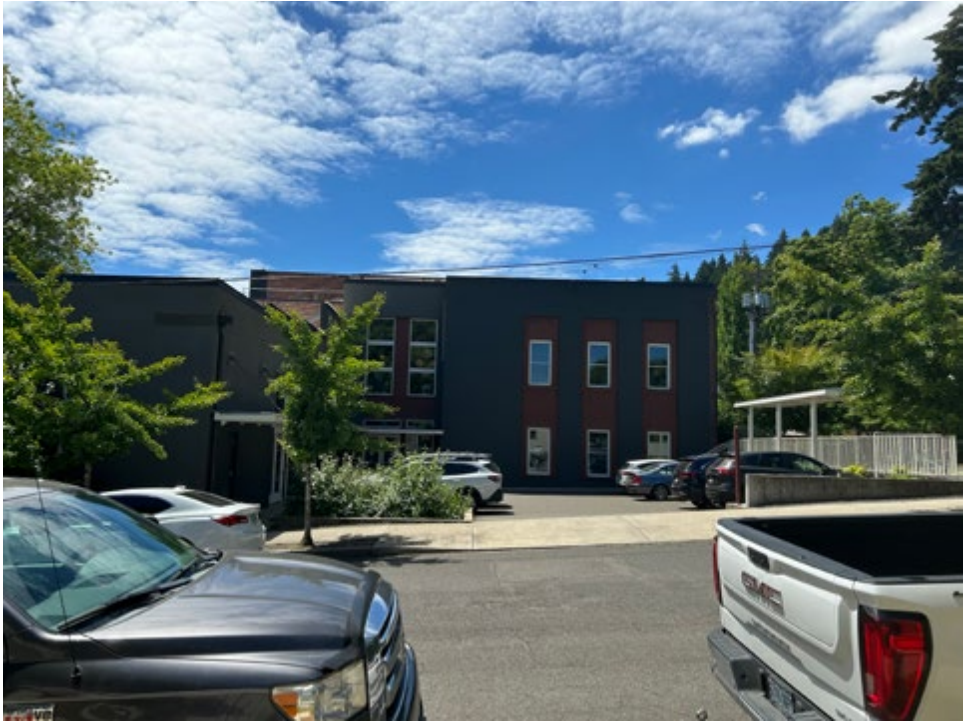
D) Porter Street Frontage - Facing South
