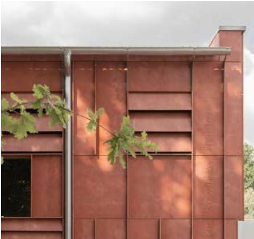
COMPOSITE WOOD FIBER AND CEMENT PANEL
