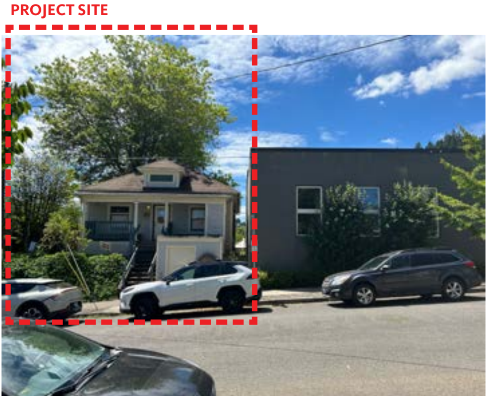
C) Porter Street Frontage - Facing South
