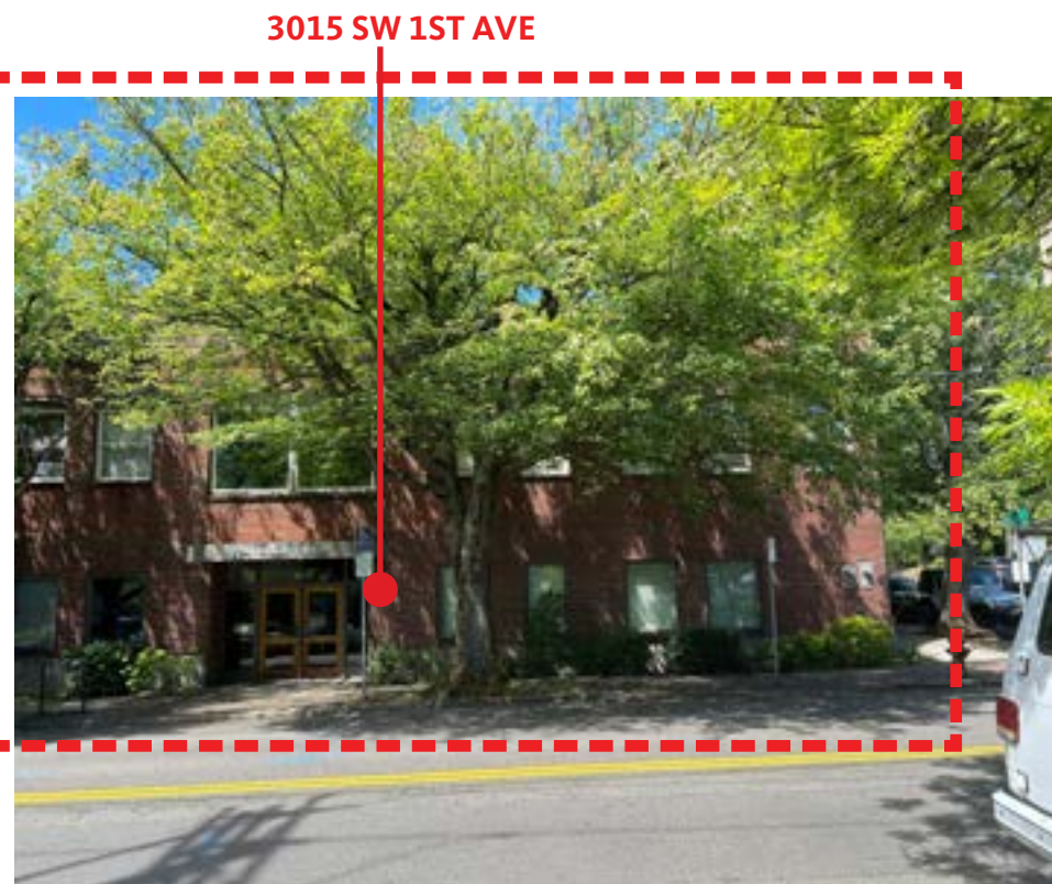
D) SW 1st Ave. Frontage - Facing West
