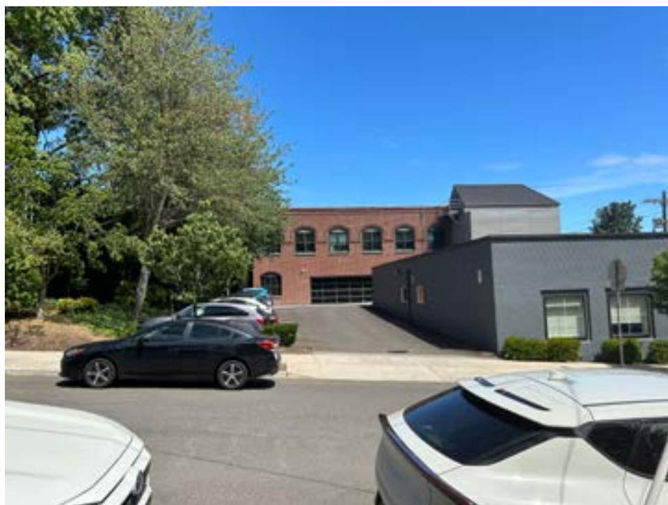
C) Porter Street Frontage - Facing North
