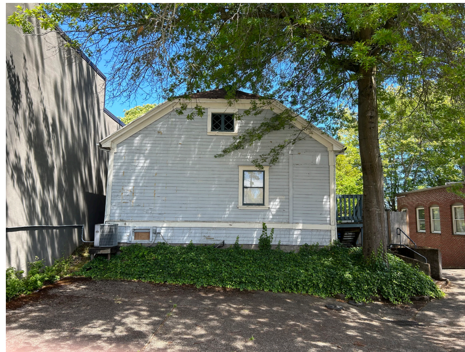
Existing on site Parking / outdoor space. - D
