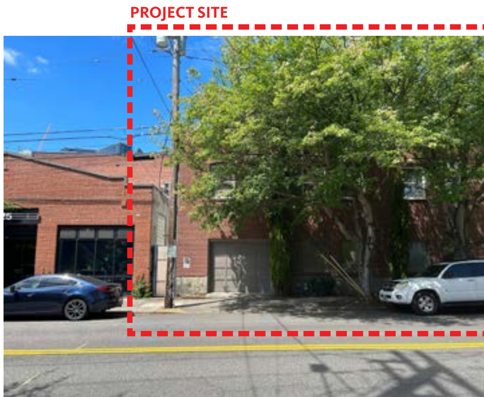
C) SW 1st Ave. Frontage - Facing West
