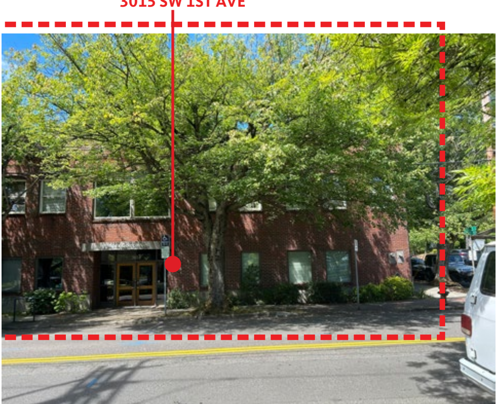
D) SW 1st Ave. Frontage - Facing West
