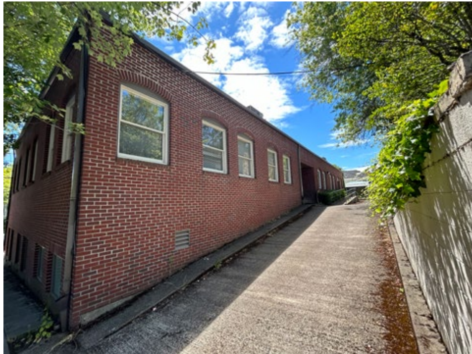
A) Existing on-site Parking Access - Facing South
