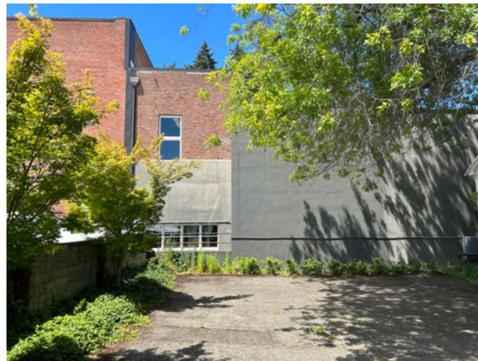
D) Existing on-site Parking - Facing West
