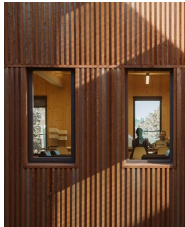
CORRUGATED METAL SIDING
