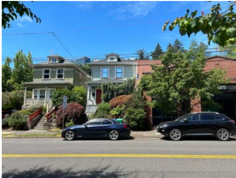
A) SW 1st Ave. Frontage - Facing West
