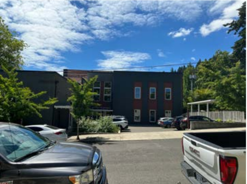
D) Porter Street Frontage - Facing South
