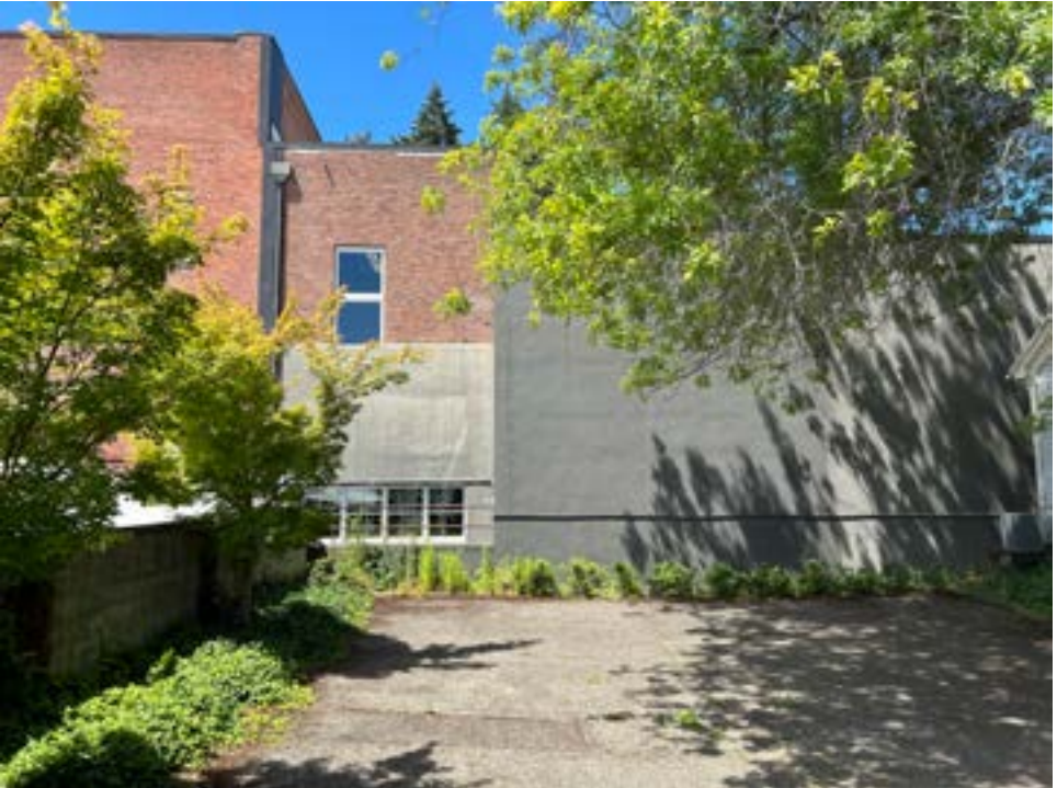
D) Existing on-site Parking - Facing West
