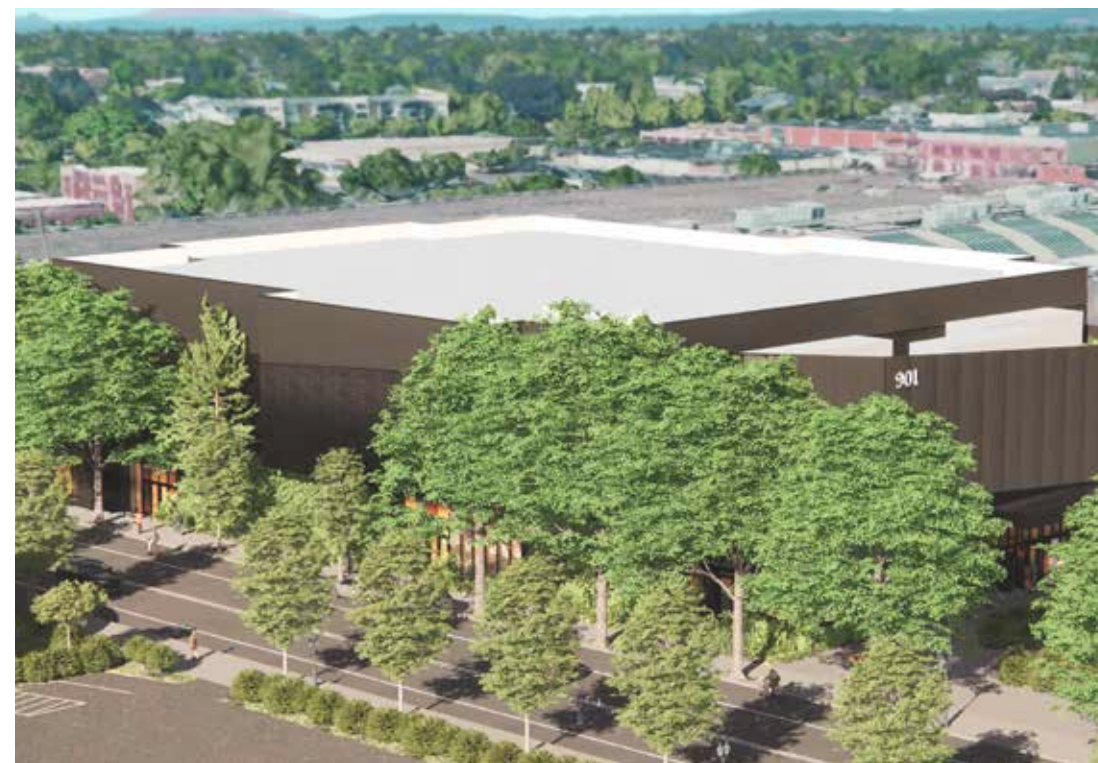
OVERALL AREAL VIEW
