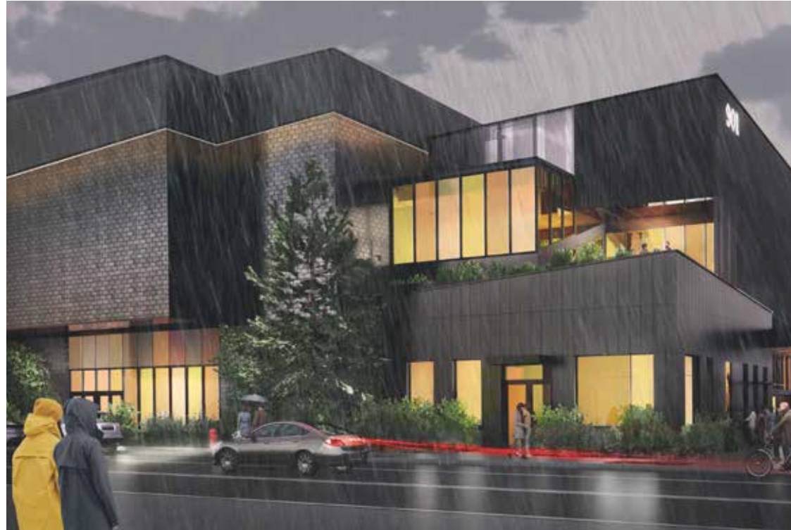
9TH AVE SOUTHWEST CORNER - ACROSS STREET VIEW
