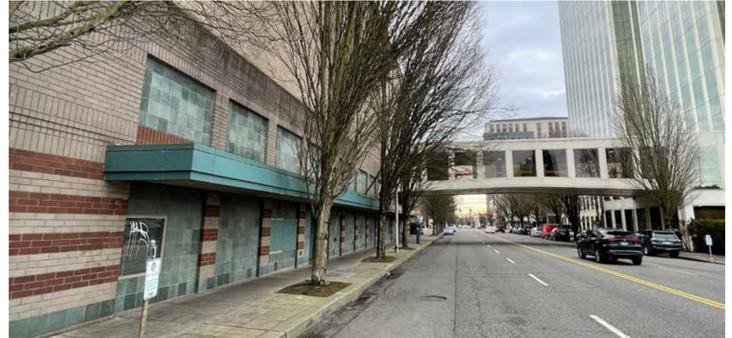
West Facade from NE 9th Ave with Existing Skybridge - Looking South
