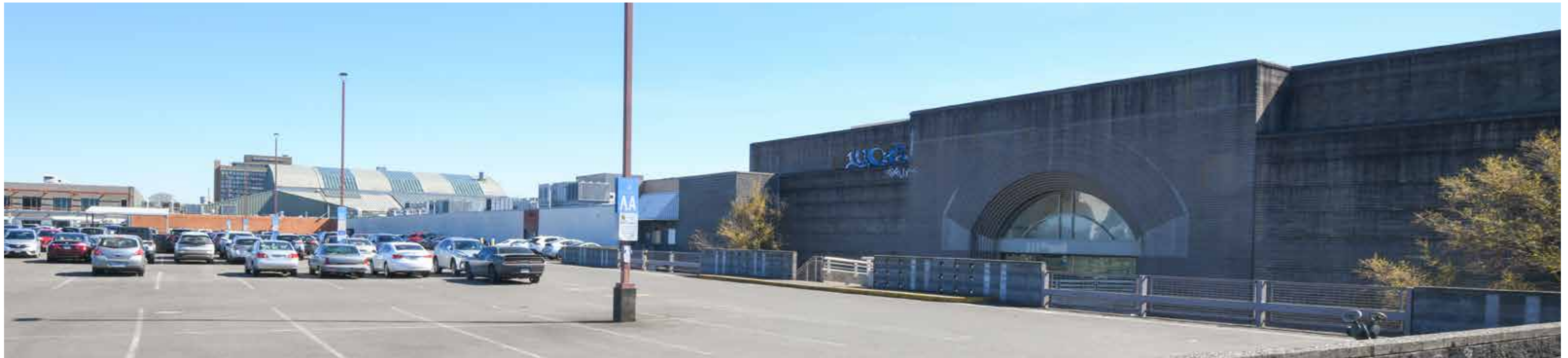
North Facade from 3rd Floor Parking Structure - Looking Southeast
