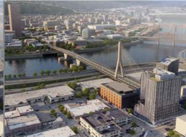
CS3- Inverted-Y tower
