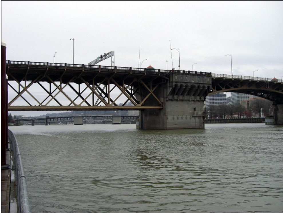
Photo 5 of 6: (OR_MultnomahCounty_WillametteHwyBridgesMPD_BurnsideBridge_0005) Upstream view, looking south, showing pier and bascule detail (Morrison Bridge in distance)
