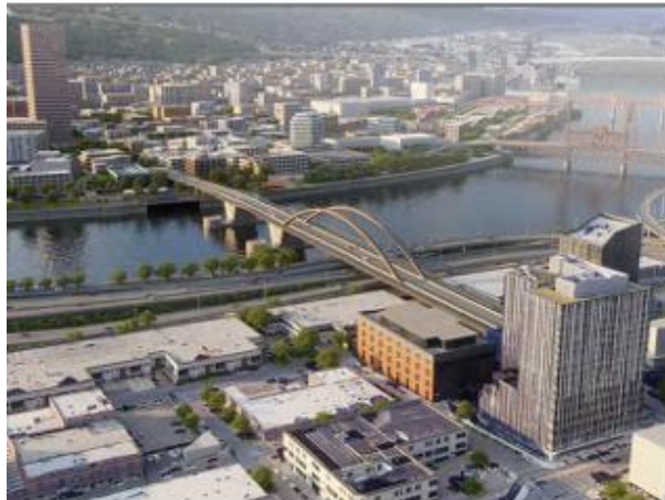
TA1-Unbraced vertical arches
