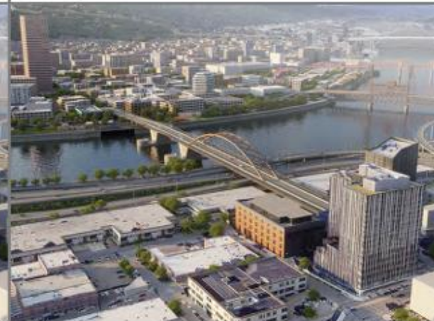
TA3- Braced vertical arches
