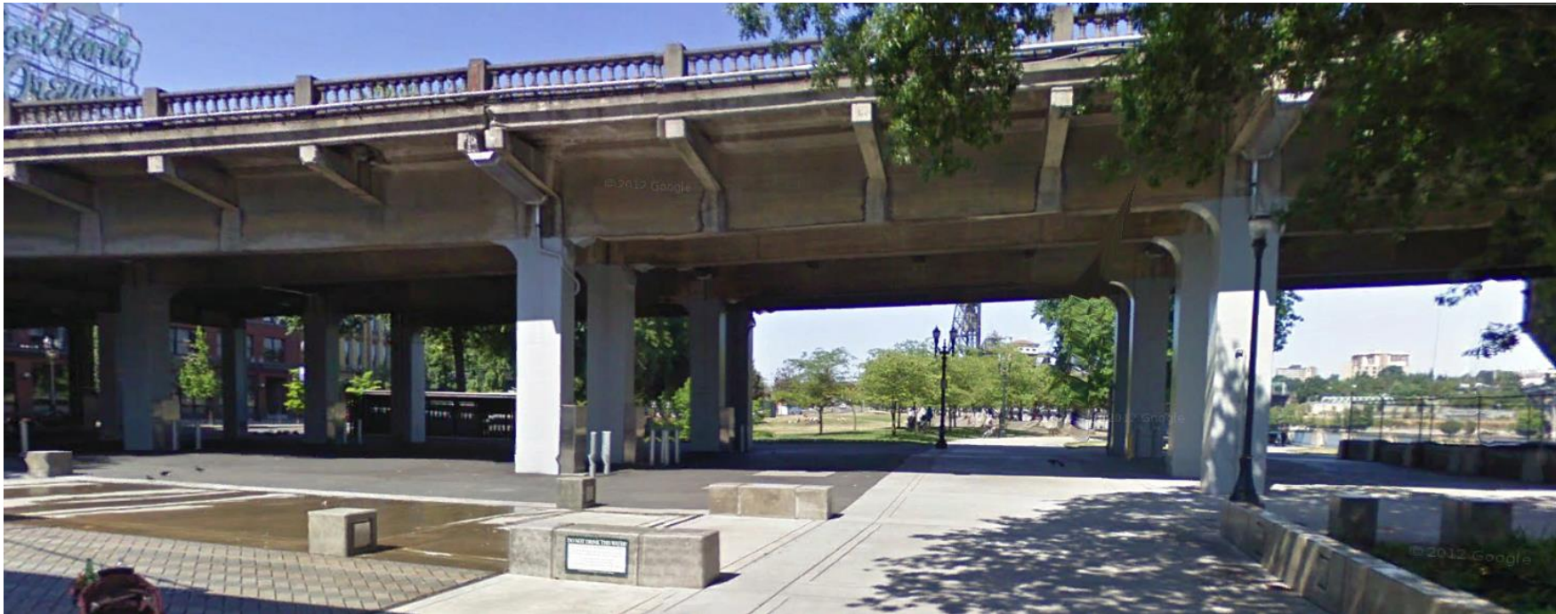
Existing condition in Waterfront Park
