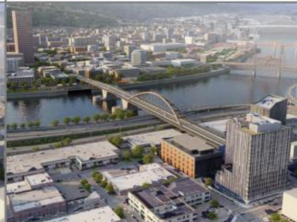
TA2-Braced basket-handle arch
