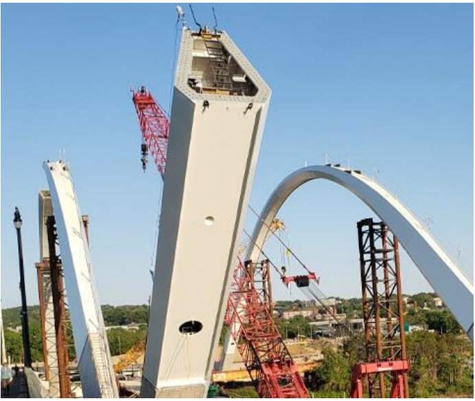
Painted Steel, fully welded variable section 6 sided parabolic arches. Sophisticated aesthetic
