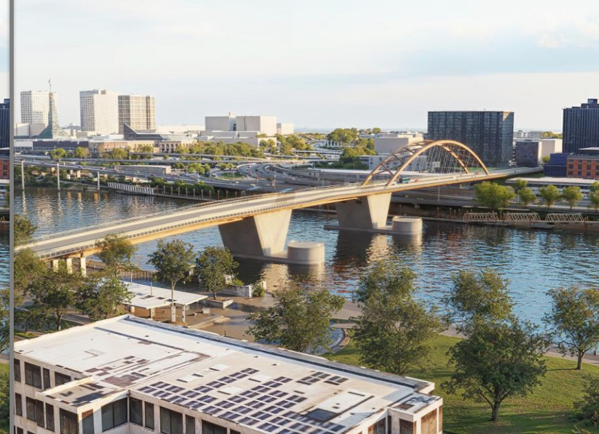
TA3- Braced vertical arches
