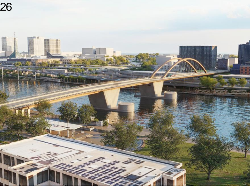
TA1-Unbraced vertical arches
