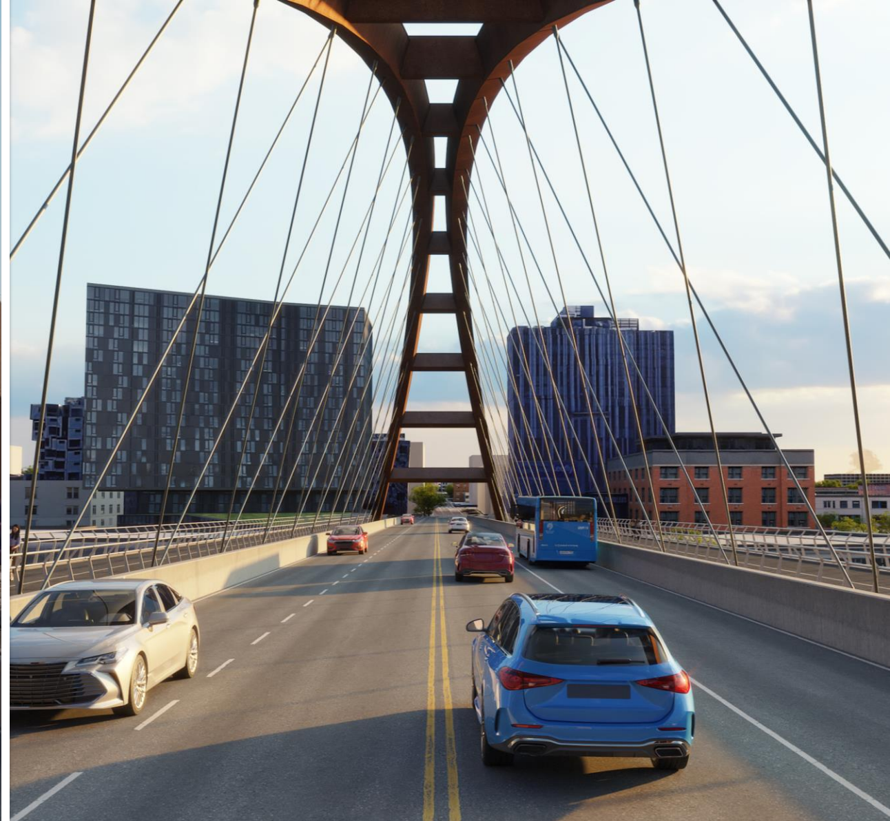
Braced basket- handle arch
