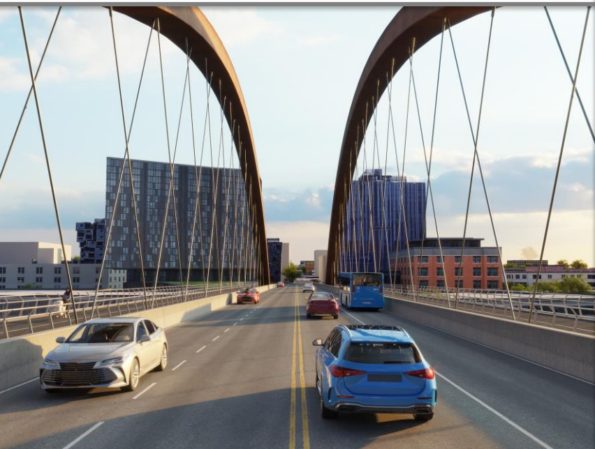
TA1-Unbraced vertical arches
