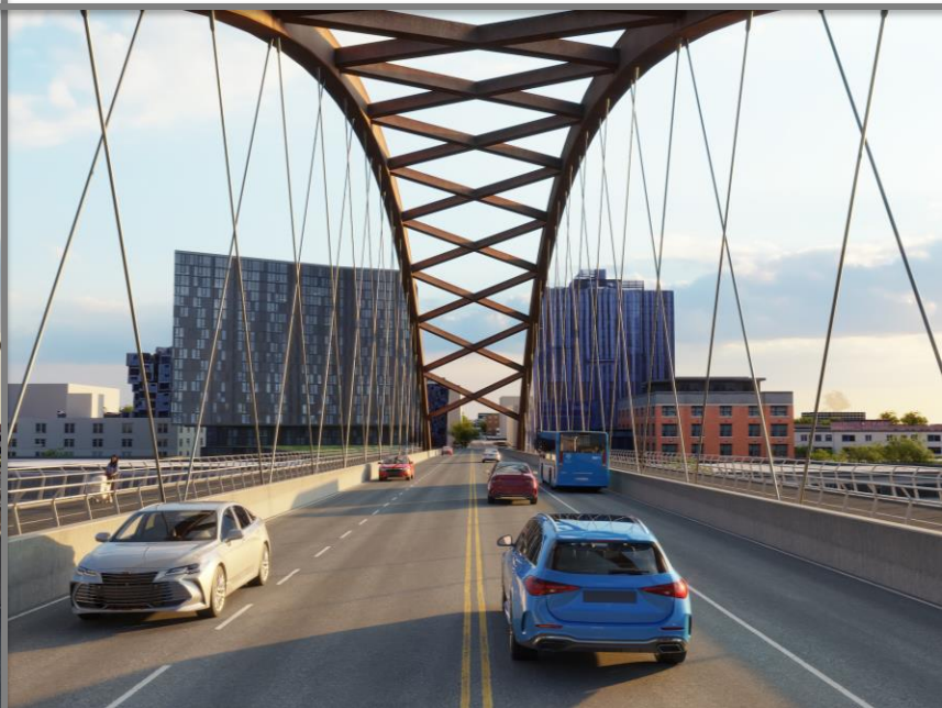
TA3- Braced vertical arches
