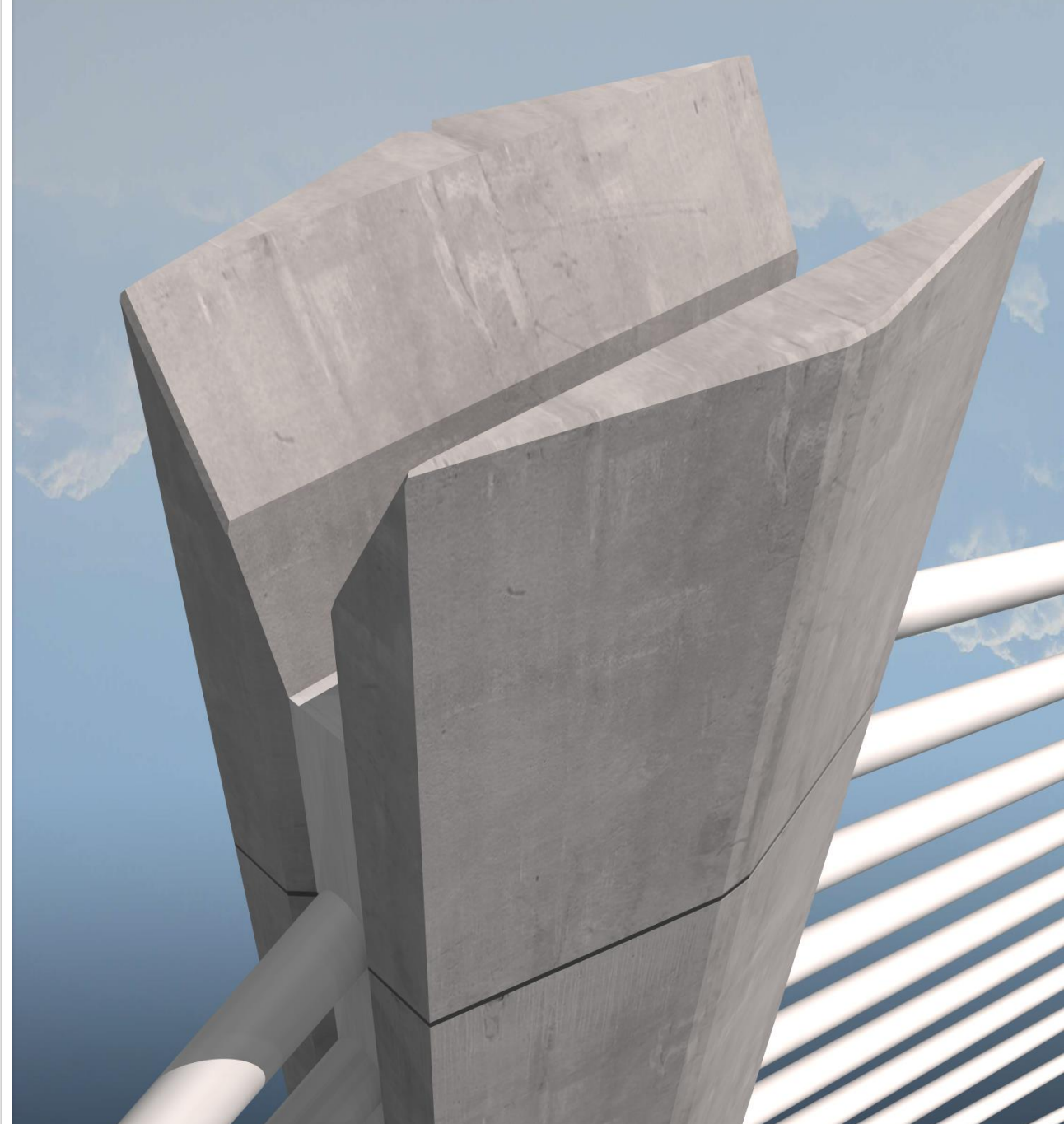
Component shaping – faceted forms make a significant difference to the perceived slenderness
