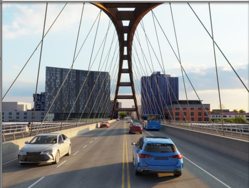
TA2-Braced basket-handle arch
