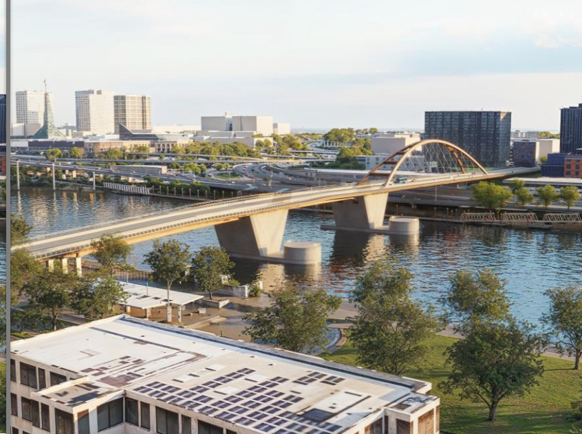
TA2-Braced basket-handle arch
