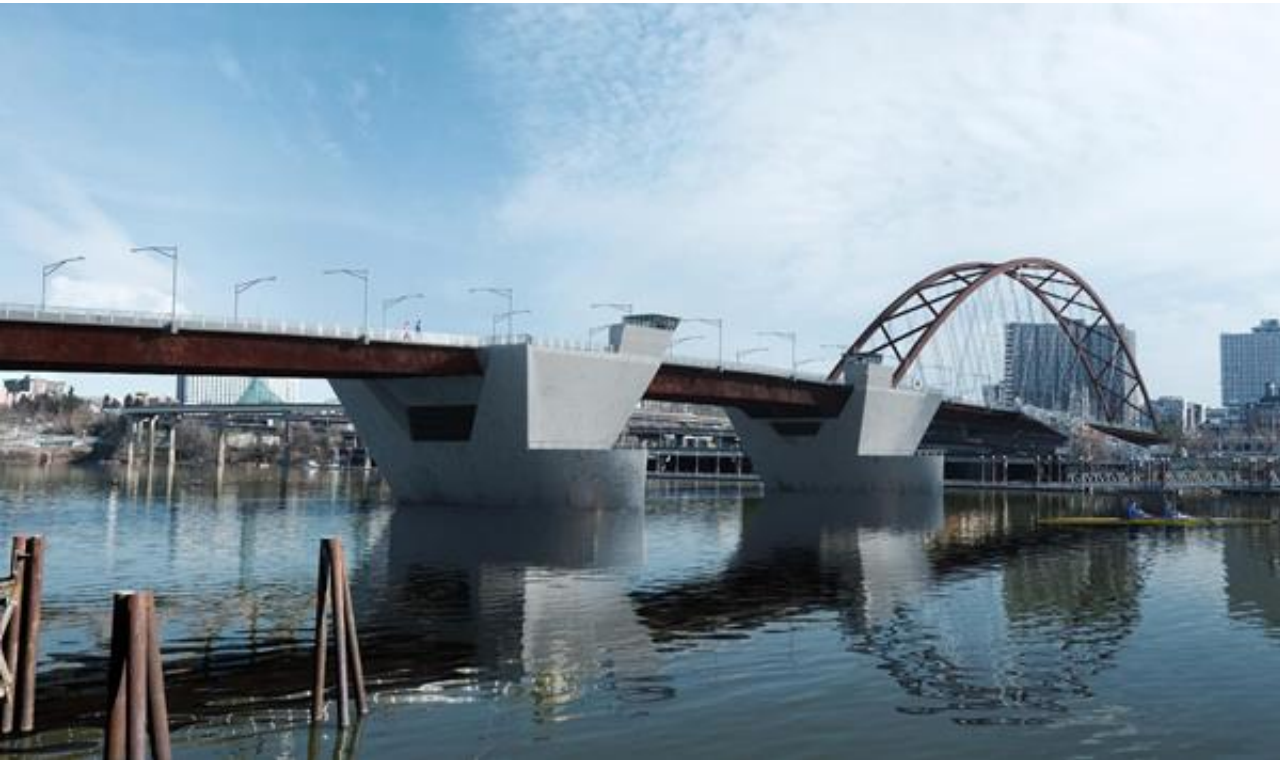
with Tied Arch for eastside long span
