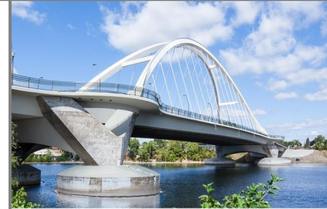
Lowry Ave Bridge, Mississippi River MN
