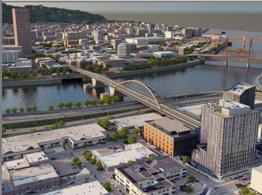
TA2 - Braced basket-handle arch
