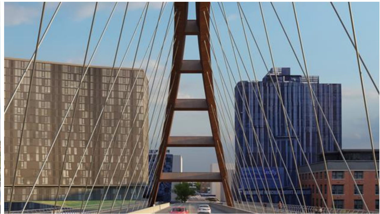
WEATHERING STEEL ARCH
