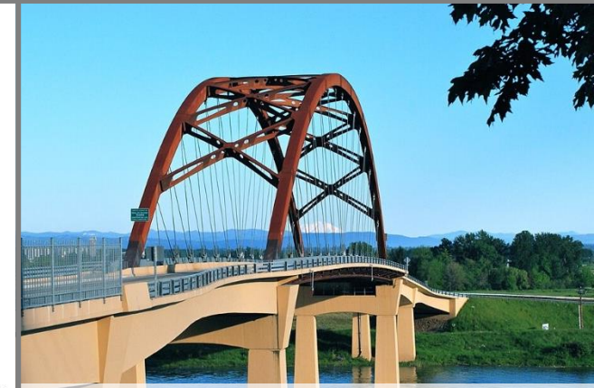
Wapato Bridge, Multnomah Channel OR
