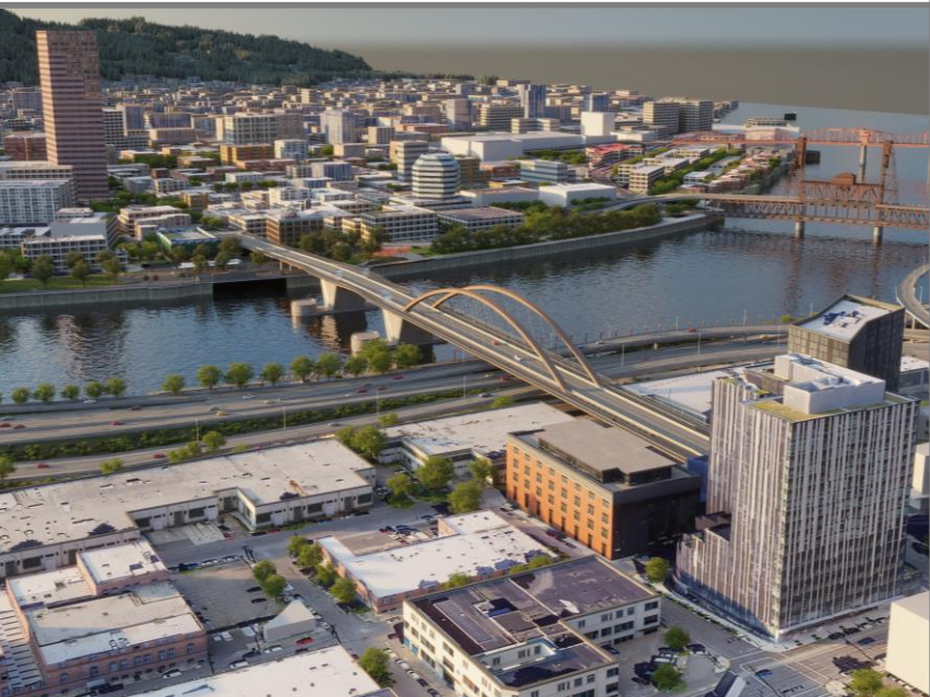
TA1 – Unbraced vertical arch
