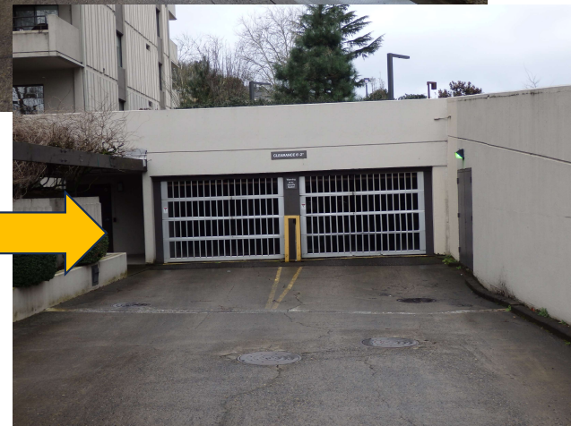
Madison Garage Entrance. One story below Plaza. The “Purple Dot”
