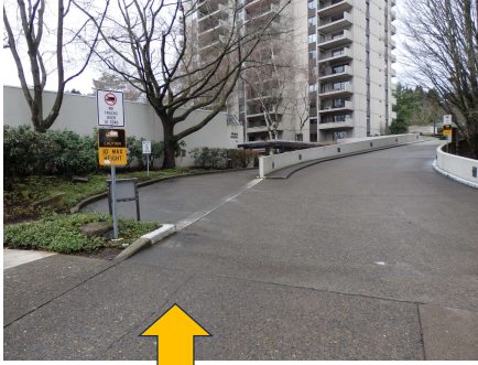
Driveway to Madison Garage Entrance and ramp to Parking Plaza from SW 1 st Ave.
