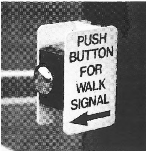
Push buttons should be marked so pedestrians know which signal is activated.
