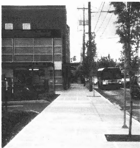
New sidewalk constructed as part of an infill redevelopment project.
