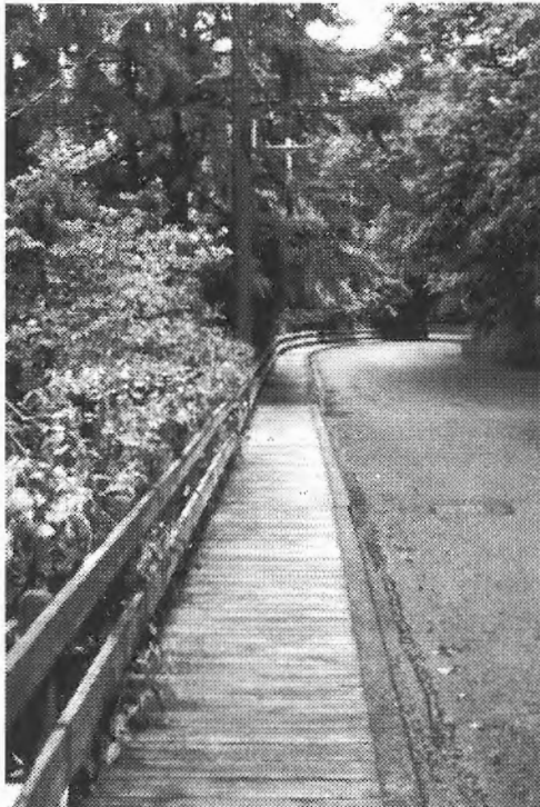
A separated alternative pathway may take the form of a boardwalk, as in this example on SW Greenway.
