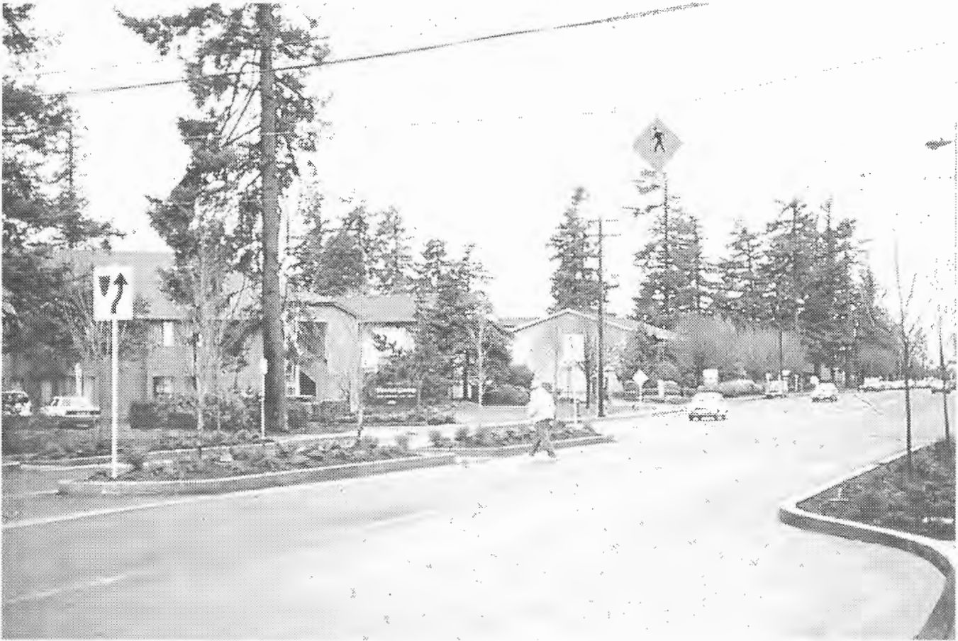
A midblock crossing improvement on a five-lane arterial street with parking. Among the crosswalk tools employed are a fully landscaped median refuge island, curb extensions and ladder pavement markings.
