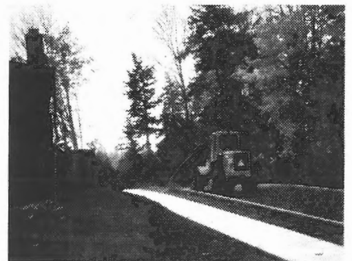
A new sidewalk constructed as part of a Local Improvement District project.
