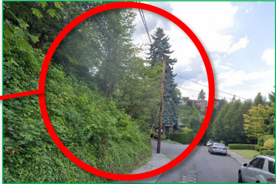
Large slope that should be studied
