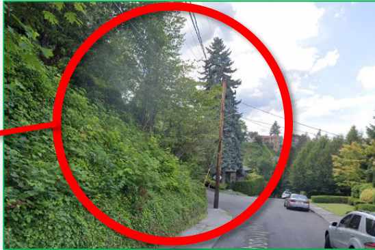
Large slope that should be studied
