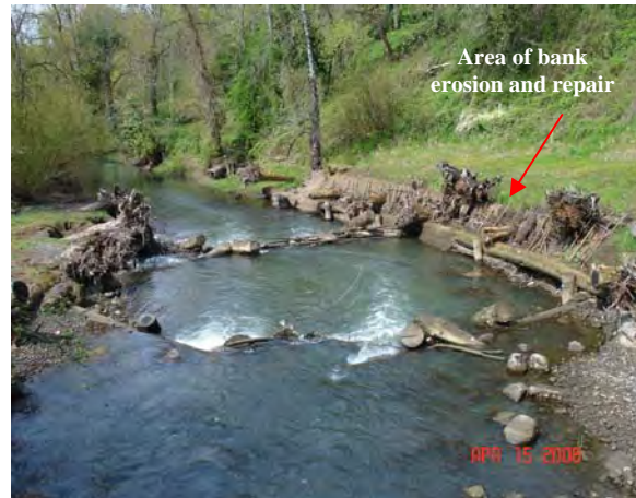
Photo 6: Tideman Johnson; erosion at lower extent of project began shortly after project completion on right bank. Willow stakes were place in the bank to prevent further erosion.
