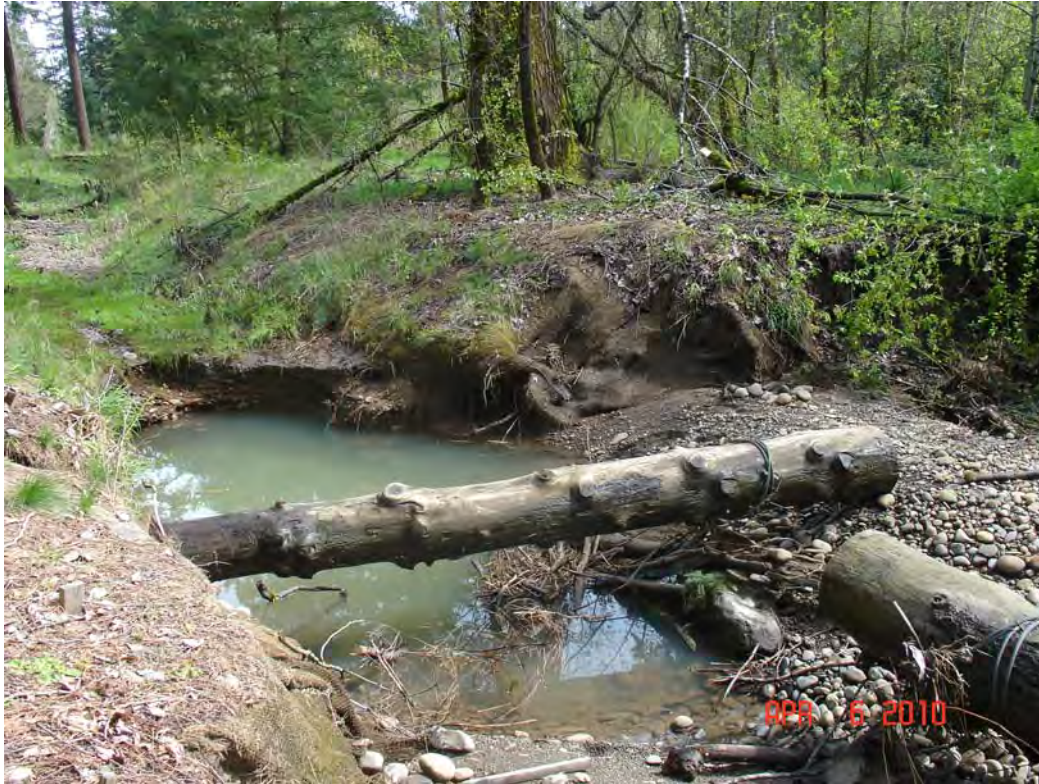
Photo 7: Scour hole at Tideman Johnson Park, in lower overflow channel.
