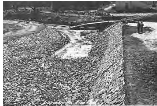
Photo 1: From 1931 – 1935, the Federal Government widened, armored and rock-lined portions of Johnson Creek as part of the WPA, in efforts to mitigate flooding.
