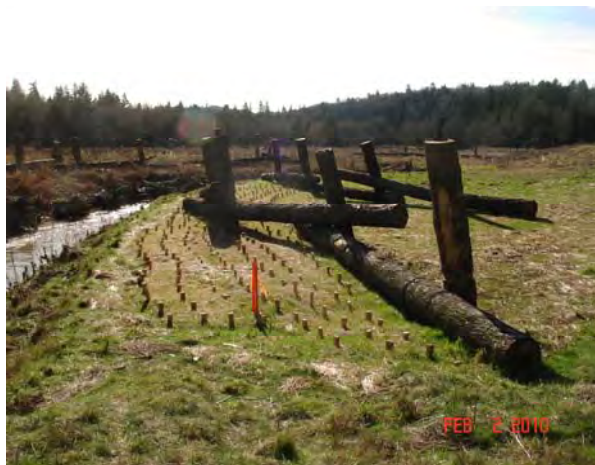
Photo 24b: Schweitzer Natural Area. Scour hole repair.
