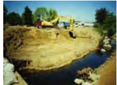
Floodplain reconnection and revegetation at Brookside (1997)
