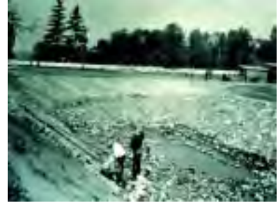
WPA rock lining and channelization (1930s)
