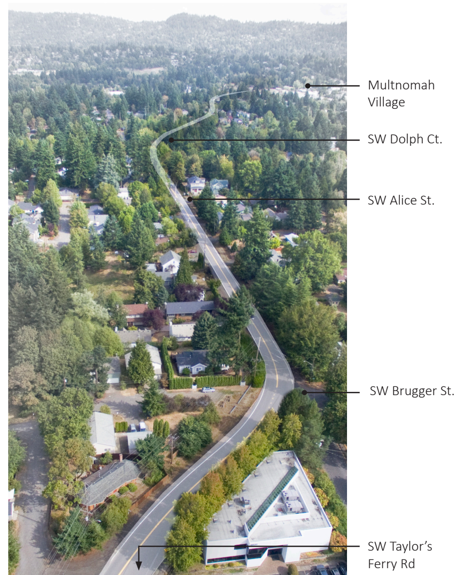
Garden Home Segment Capitol Highway Corridor Overview
