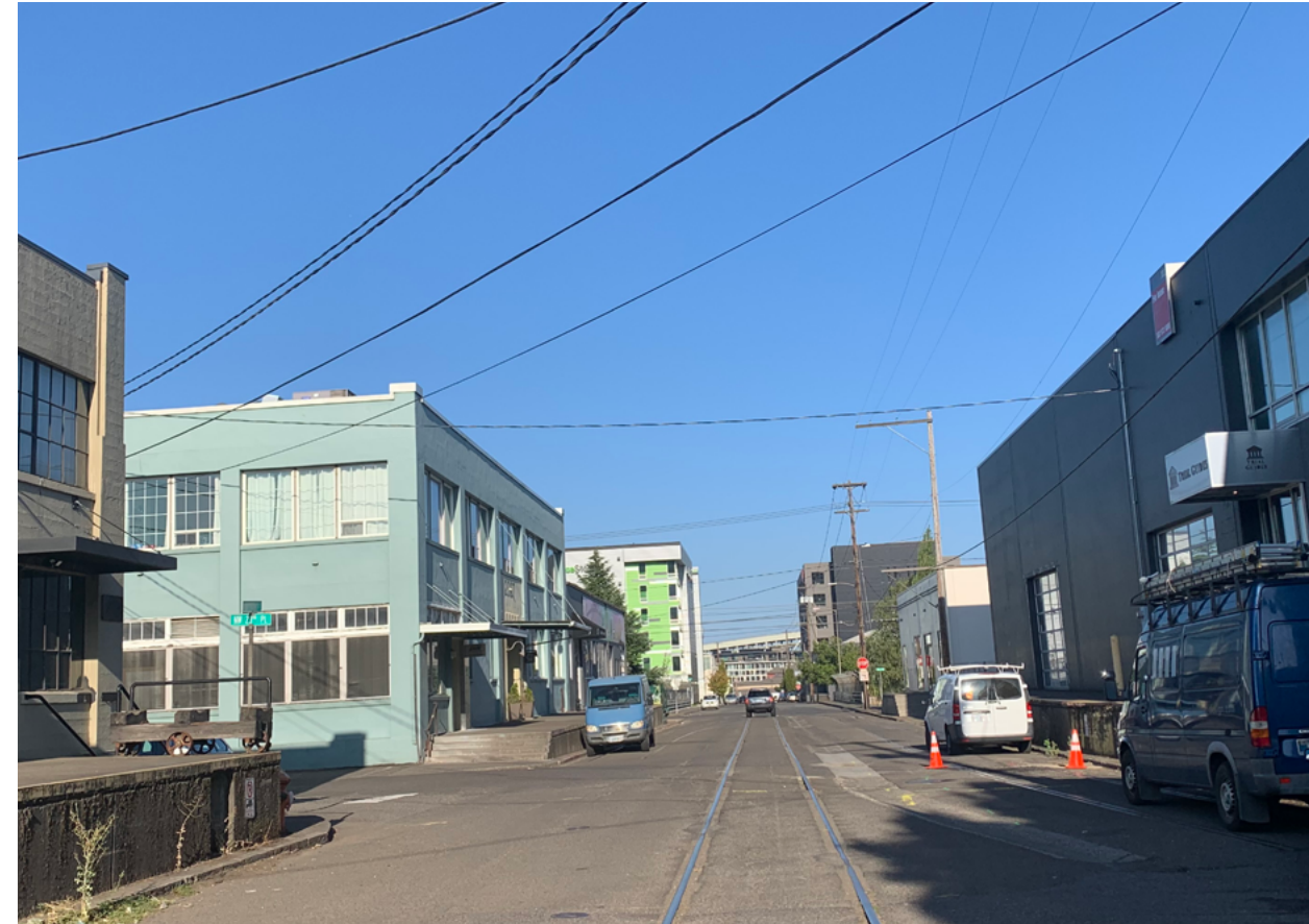
EXISTING CONDITIONS ON NW YORK STREET WEST OF NW 23RD AVENUE
