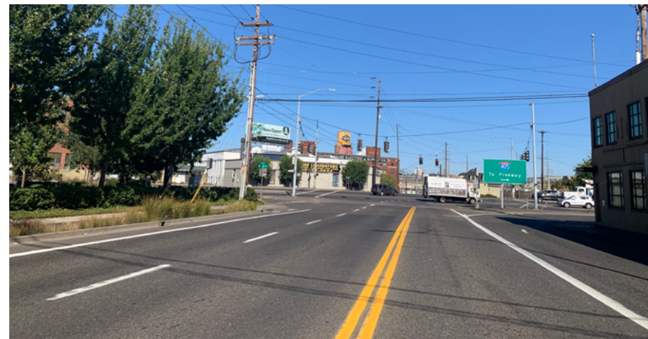
NW NICOLAI ST TOWARD NW 23RD AVE/US-30 RAMPS TODAY
