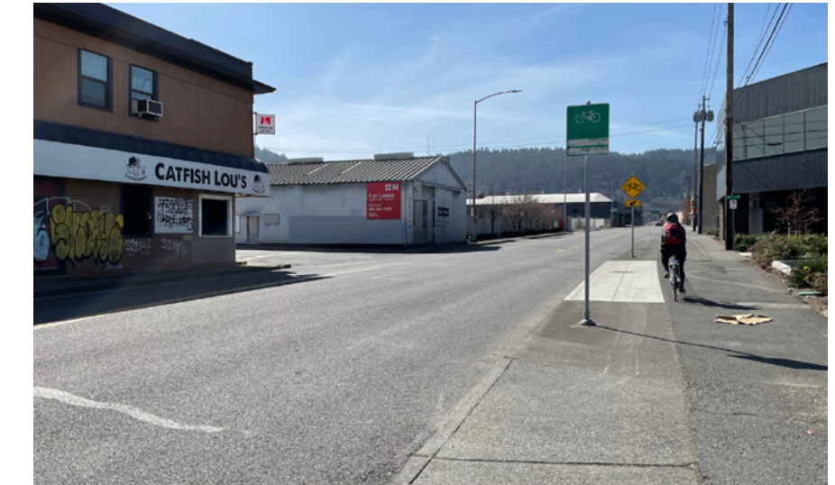
NW NICOLAI STREET WITH OLD RAIL SPUR ON RIGHT TODAY
