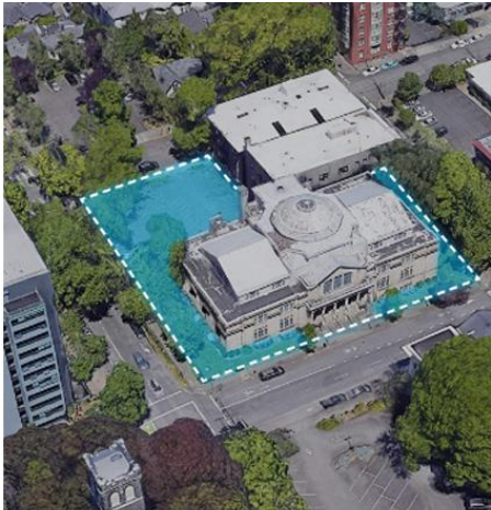
Aerial of Proposed Project Site looking NE
