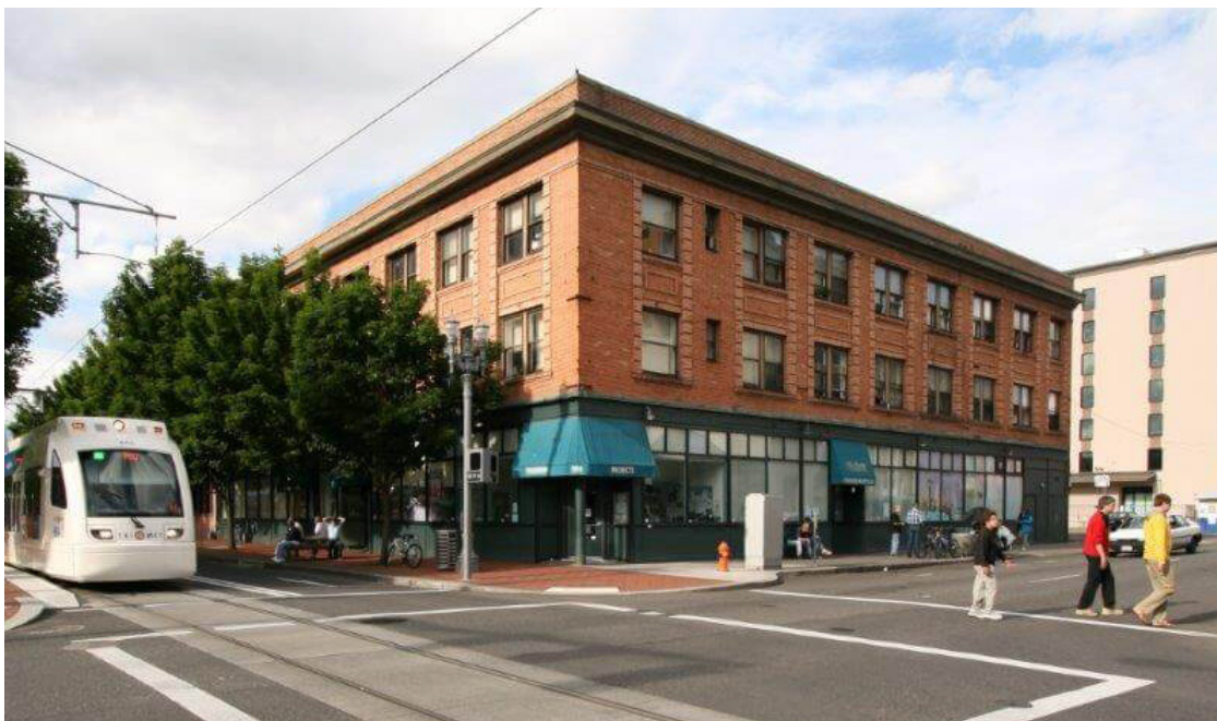
Central City Concern's Medford Hotel, which comprises 61 SRO units. It is a URM building.
