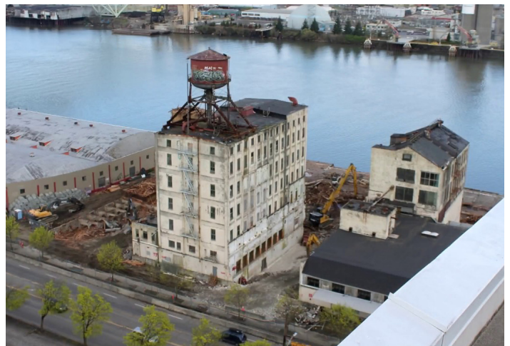
Centennial Mills, current condition
