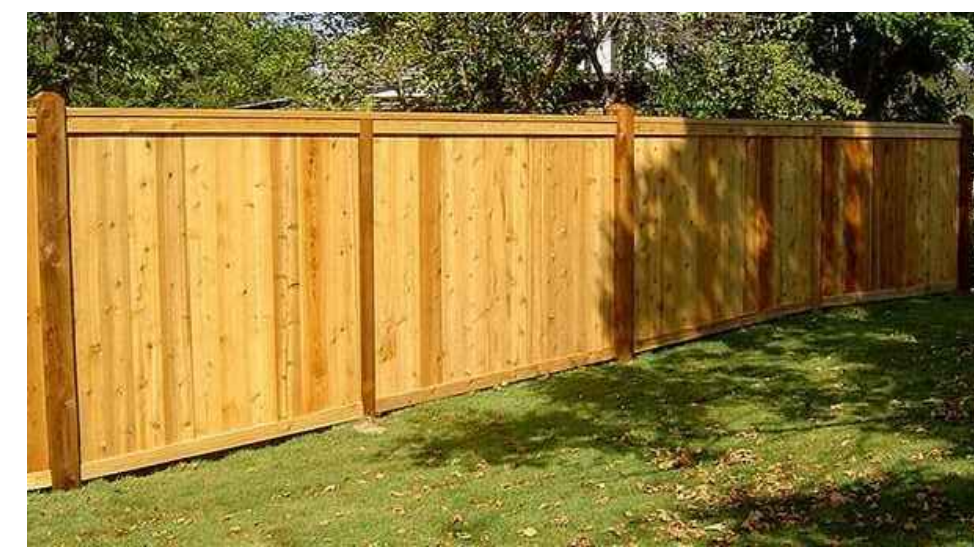
6' HIGH 100% FULLY SITE-OBSCURING WOOD FENCE
