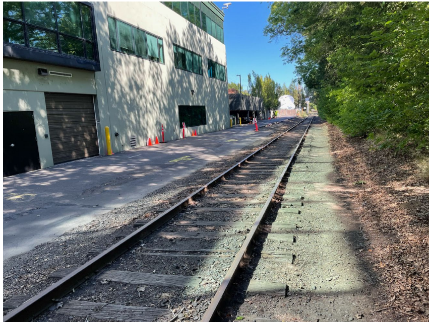
Looking north, at eastern rail ROW
