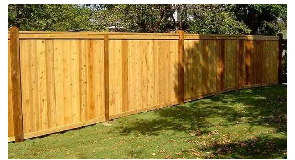
6' HIGH 100% FULLY SITE-OBSCURING WOOD FENCE
