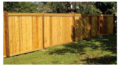
6' HIGH 100% FULLY SITE-OBSCURING WOOD FENCE
