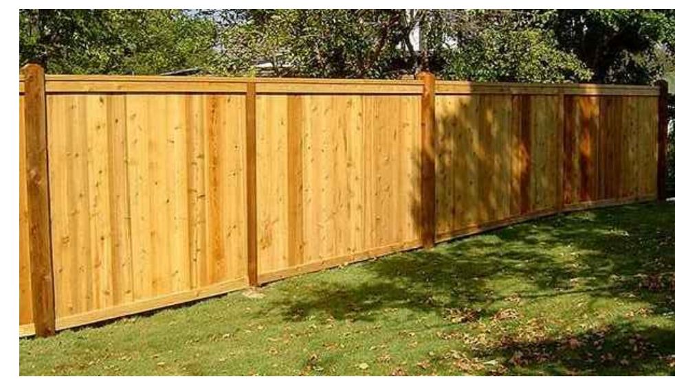
6' HIGH 100% FULLY SITE-OBSCURING WOOD FENCE
