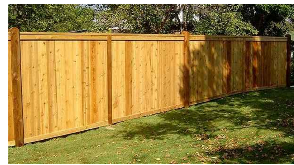
6' HIGH 100% FULLY SITE-OBSCURING WOOD FENCE
