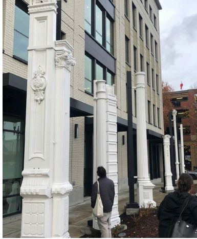
Cast Iron installation on Natio
