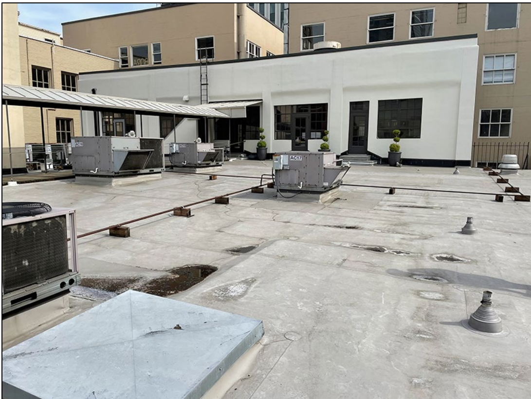
Photo 2 of 12: OR_MultnomahCounty_AlderwayBuilding_0002 Roof and south elevation of penthouse, camera facing north.
