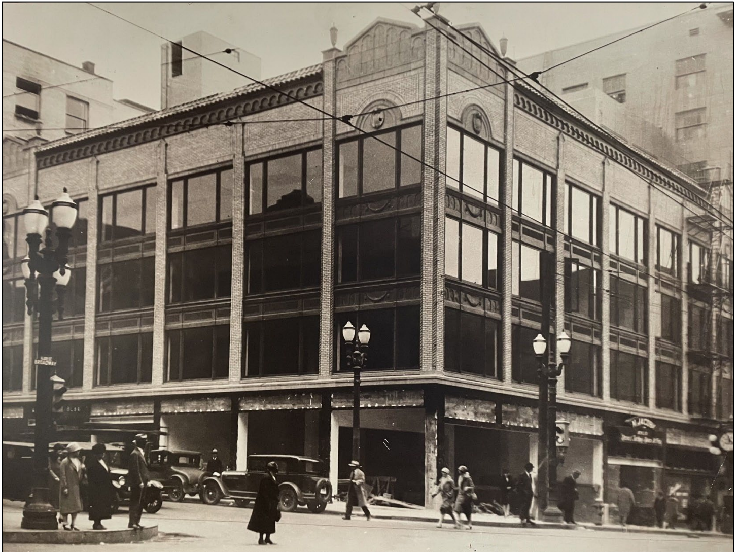
Figure 15: September 30, 1928 Construction Photo of the Alderway Building (Oregon Historical Society)
