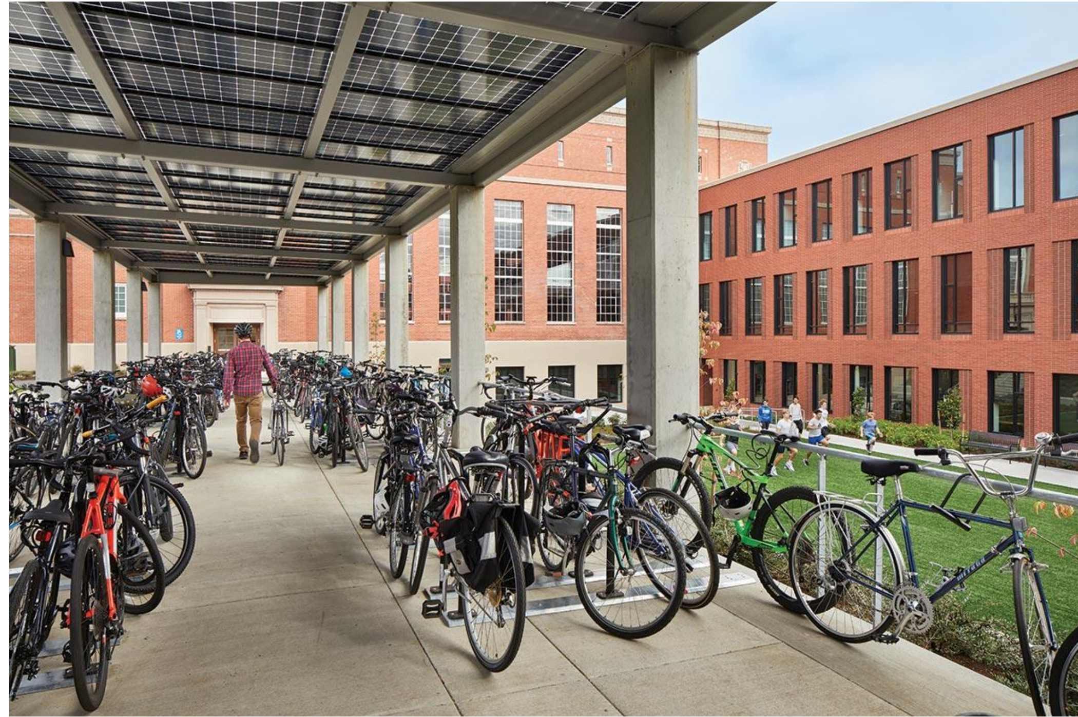
Grant HS Concrete structure with photovoltaic roof On Park-Side of School, not visible from street Unsecure 144 covered 76 uncovered 220 spaces
