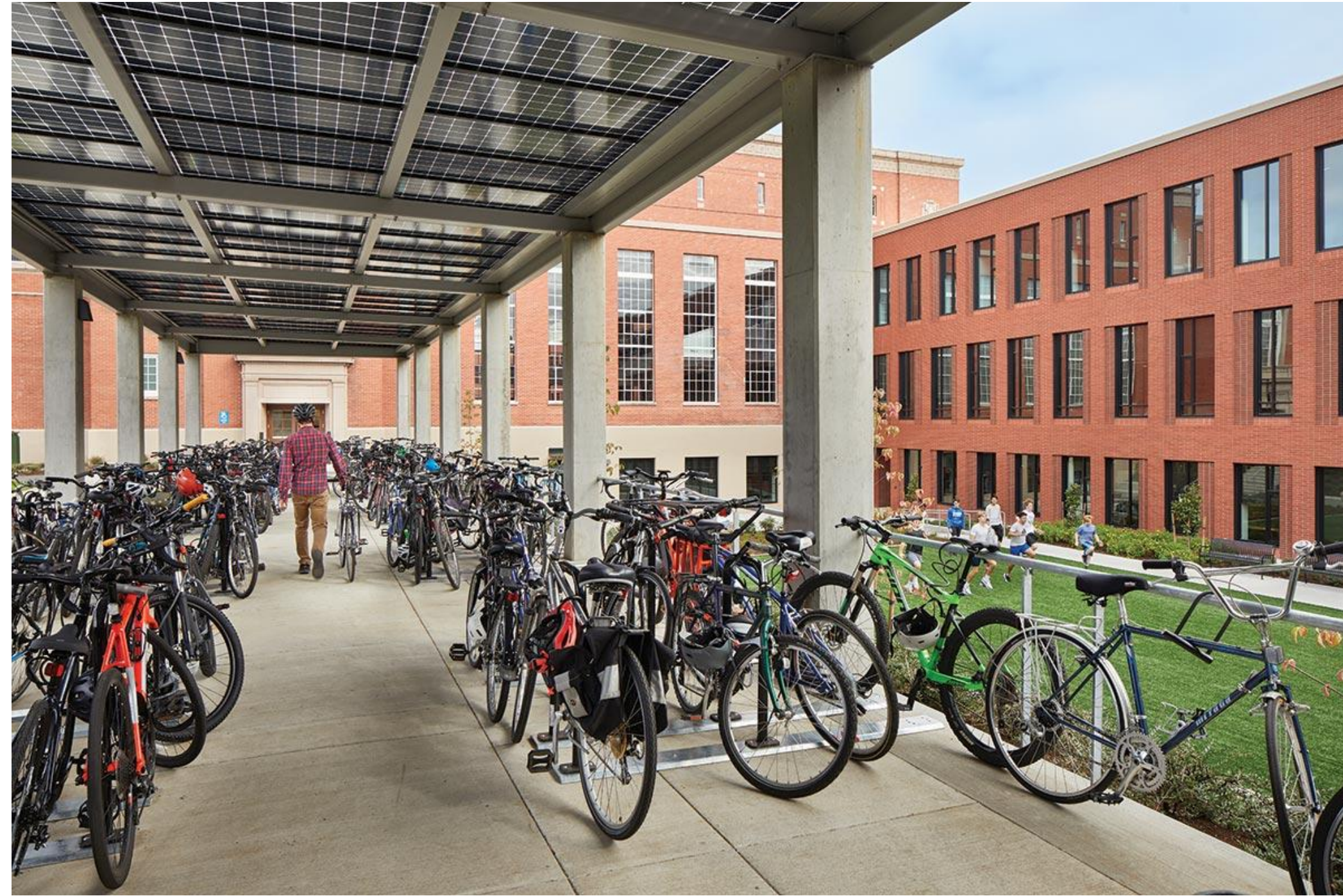
Grant HS Concrete structure with photovoltaic roof On Park-Side of School, not visible from street Unsecure 144 covered 76 uncovered 220 spaces
