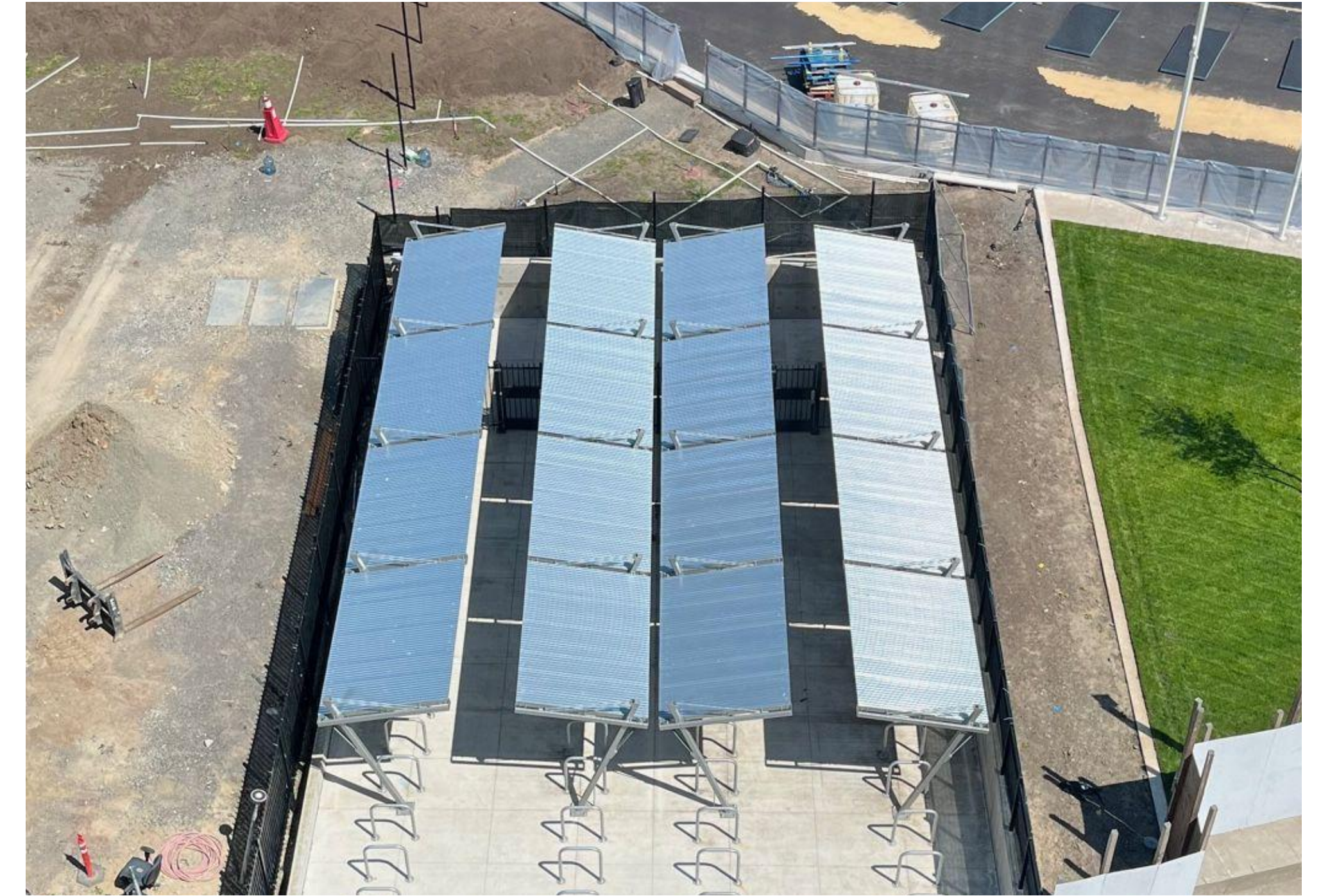
Lincoln High School Pre-Manufactured system, Dero- Visor System Visible from Street Secured behind School Fence 128 covered 24 uncovered 152 spaces
