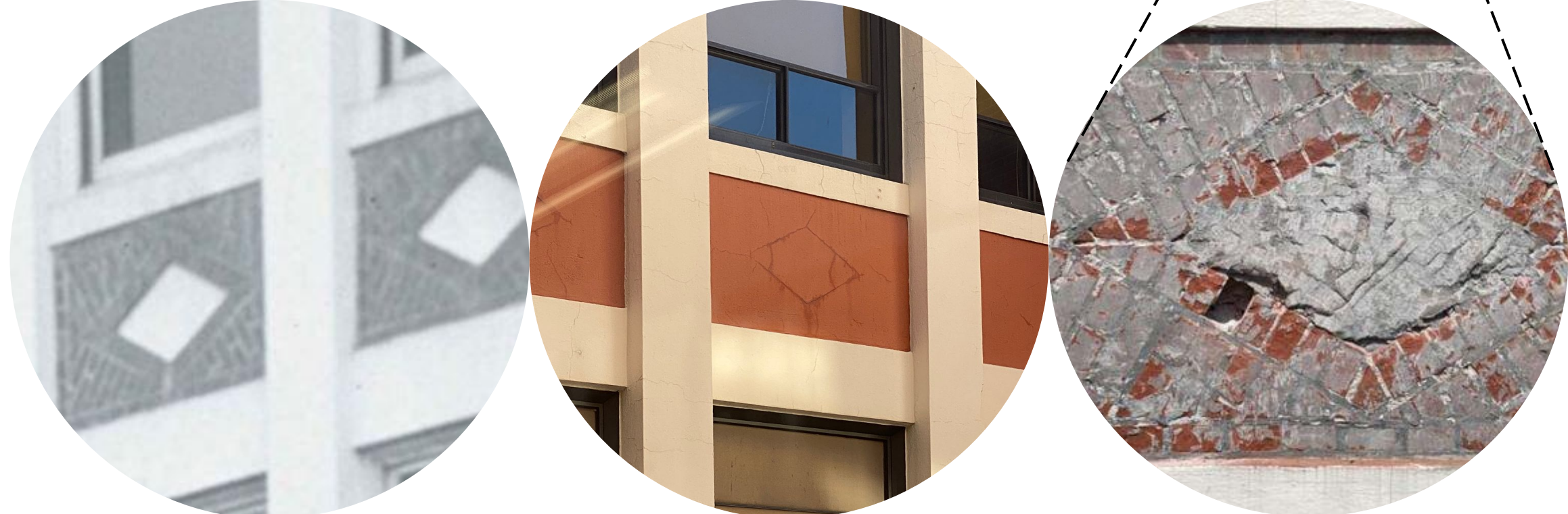
Diamond Panels between Levels B+C
