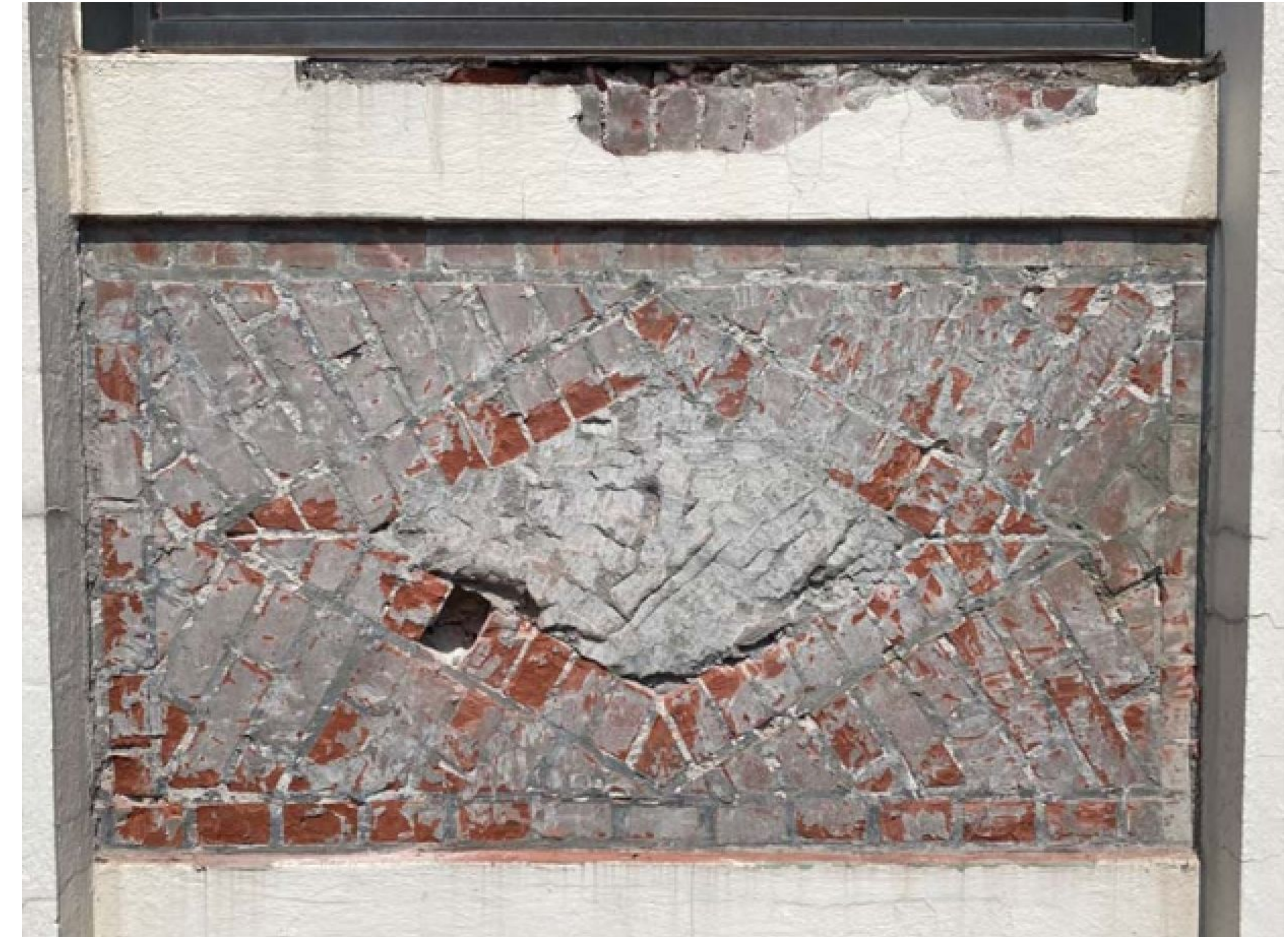
Brick after removal of plaster
