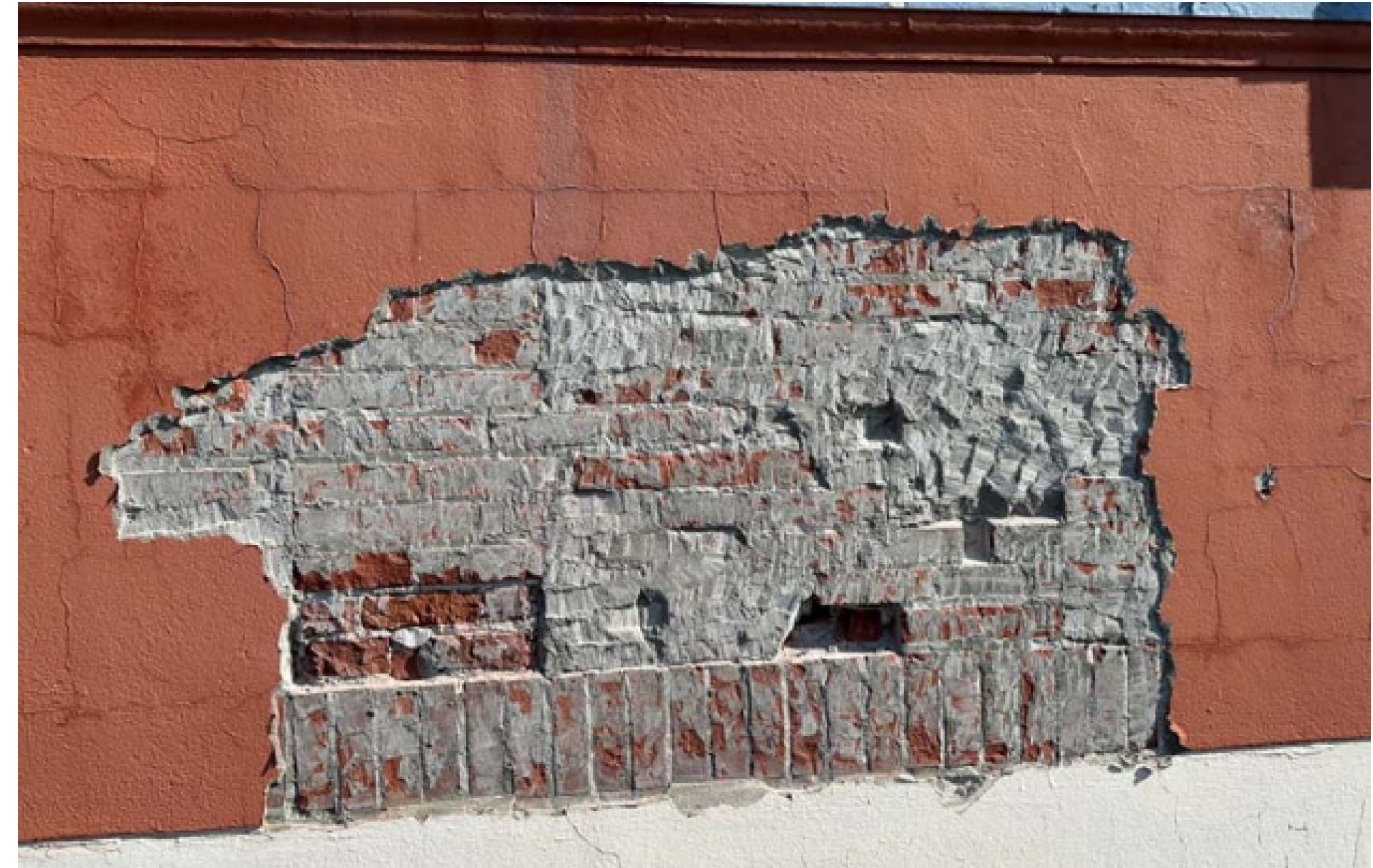
Brick after removal of plaster
