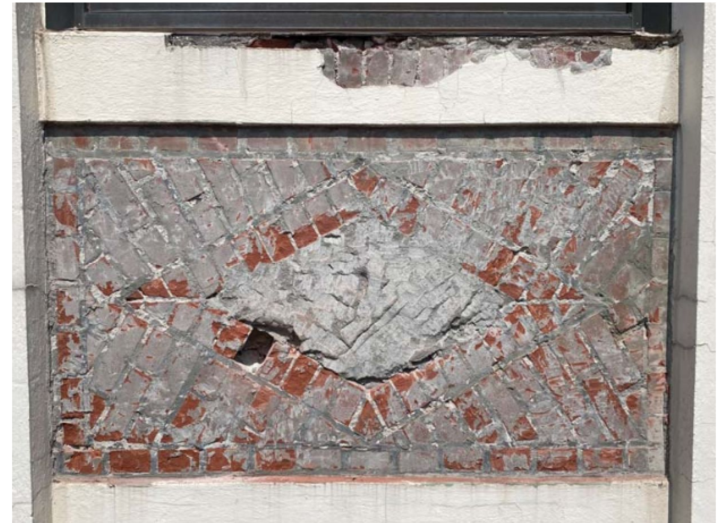
Brick after removal of plaster
