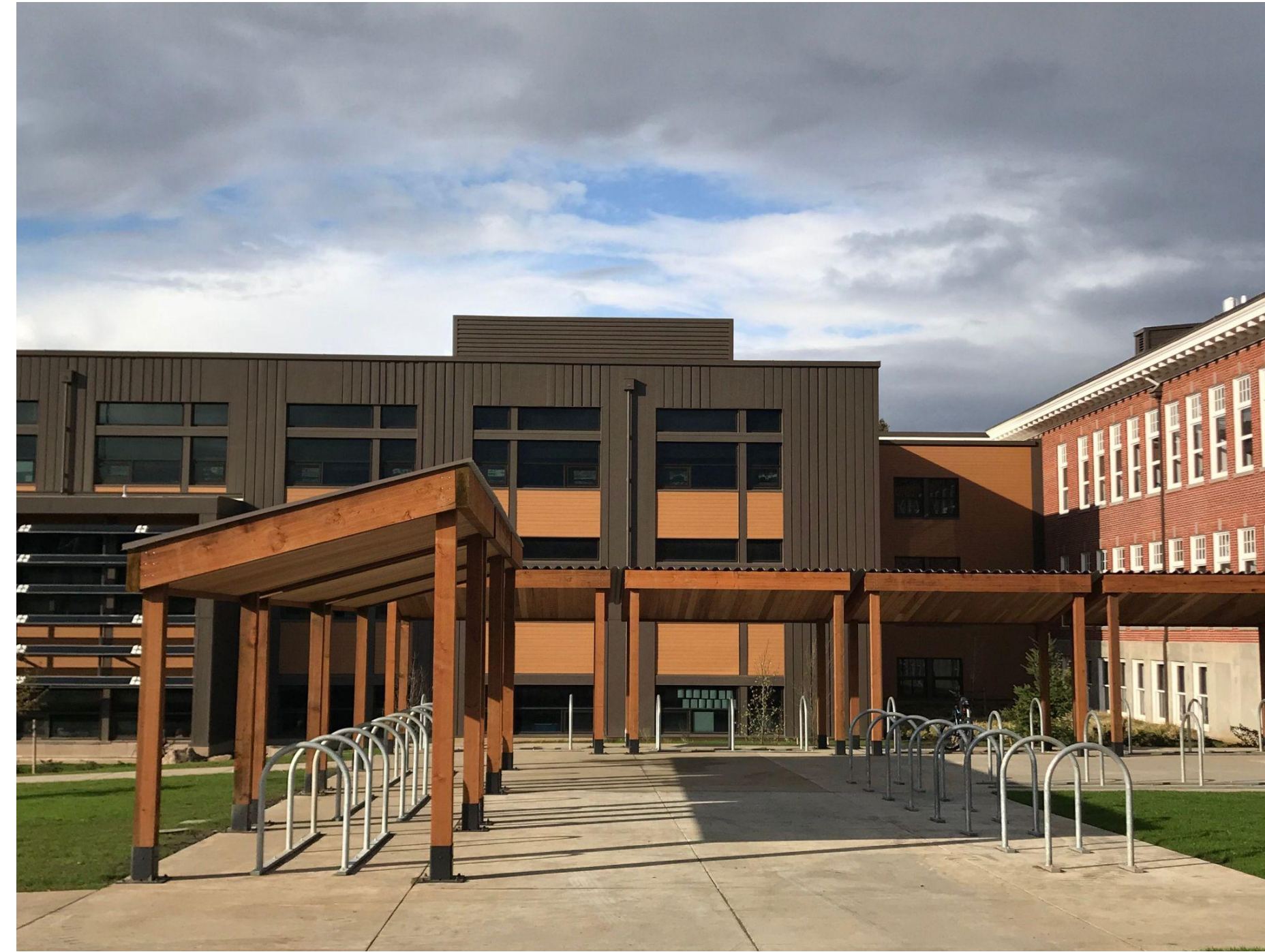
Roosevelt HS Wood Structure Visible from Street Unsecure 42 covered 58 uncovered 100 spaces
